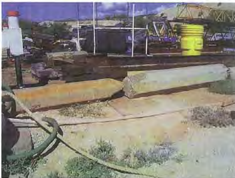
Photo 48: The shore side staging area for the Lil' Perris dry dock has a berm built from cement pillars. Plastic sheeting has been laid down against the pillars and covered with dirt, however the plastic sheeting has torn away in most areas and gaps are prevalent along the entire berm.
