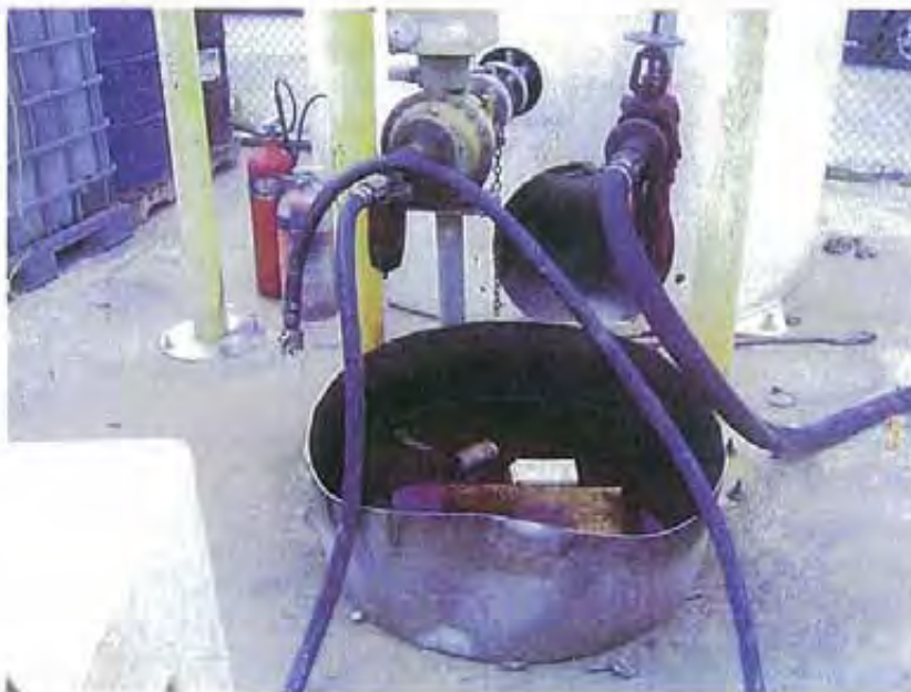
Photo 36: A drip pan for a 3,000 gallon diesel tank was observed containing diesel, open and exposed to rain fall, without secondary containment.
