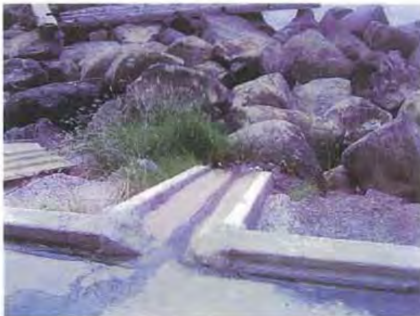
Photo 24: Another photograph of the storm water outfall for the area behind the metal working building. Wash water runoff is visible discharging down the outfall.
