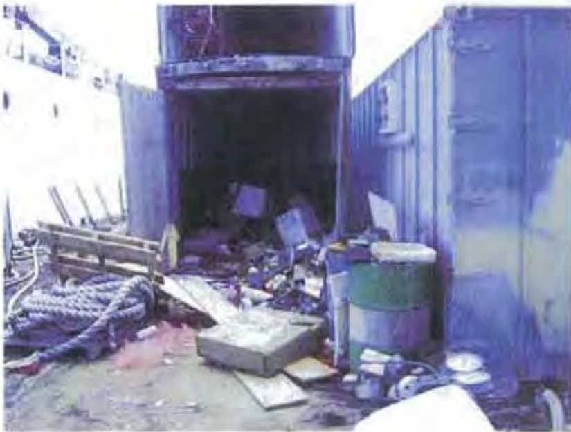
Photo 41: Debris and materials scattered on the floor of the work barge outside a storage shed. Two 55-gallon drums of oil were observed on the deck of work barge, without secondary containment.
