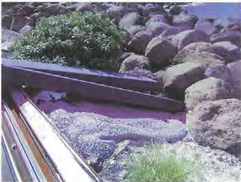
Photo 22: Evidence of concrete spillage from an on-site construction activity (possibly the construction of the concreted area itself or the berm) toward the receiving water. It is unclear if any of the concrete actually entered the receiving water. However this photo demonstrates a lack of effective best management practices utilized for the construction project by the Discharger this close to the edge of the receiving water.
