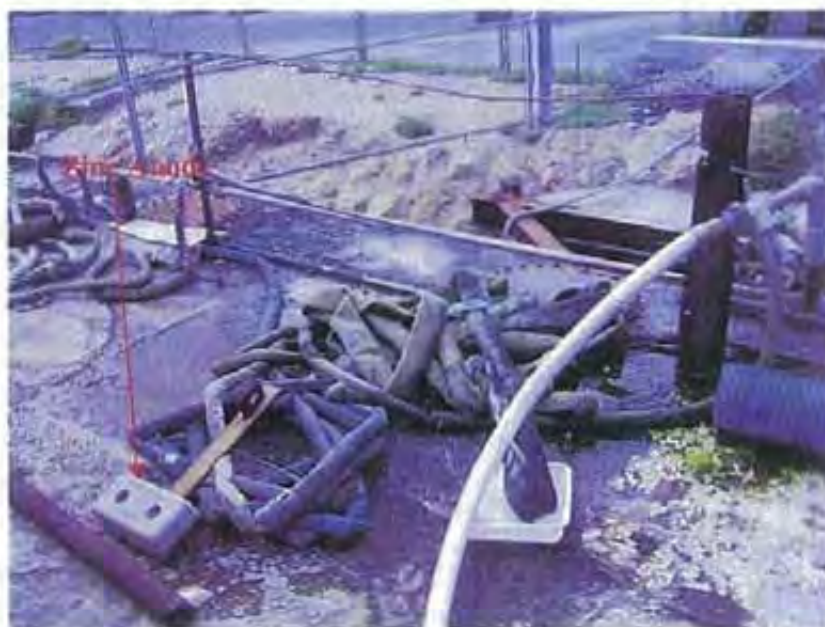
Photo 43: These water lines are used to supply the workers with potable water as they work on-board vessels. The line/hose hook ups were observed leaking and draining over the edge of the work barge. Also pictured above is a zinc anode on the deck of the work barge, near the draining water.
