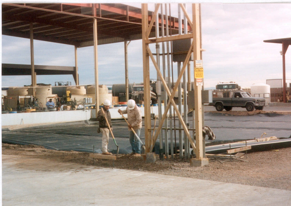
Final preparations on liner prior to covering
