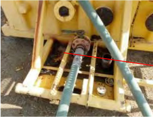
Olympus Stylus 8000, Photo #56; View of the leachate collection frac tank at WMU 34, facing east. Note the stains around the valve area and on the ground.
