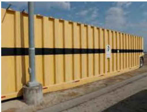
Olympus Stylus 8000, Photo #55; View of the leachate collection frac tank at WMU 34, facing northeast.
