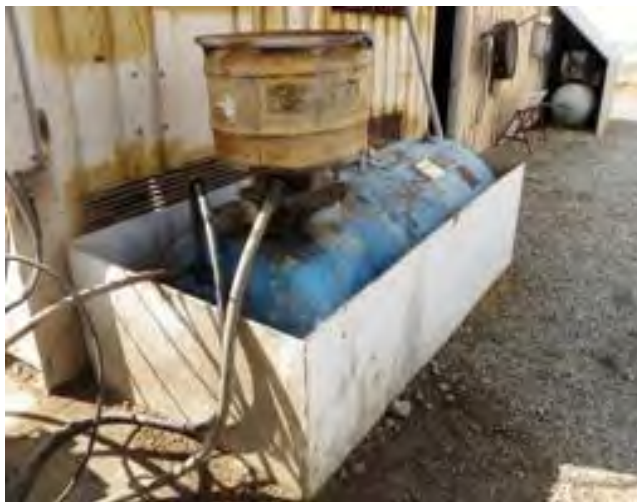
Olympus Stylus 8000, Photo # 50; View of the used oil storage tank at the maintenance building.
