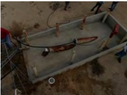
Olympus Stylus 8000, Photo #76; View of the leachate collection system at WMU 28 from the top of the leachate collection frac tank (Frac Tank 3)
