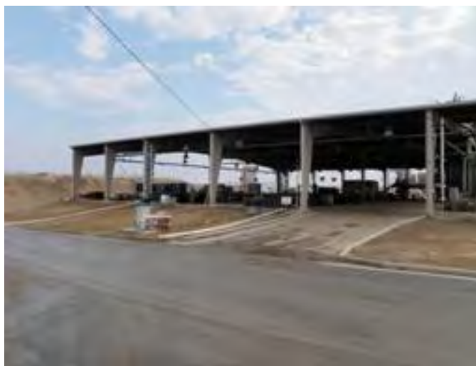
Olympus Stylus 8000, Photo #2; View of the drum storage area in the Stabilization/Treatment Unit (STU) area, facing northeast.
