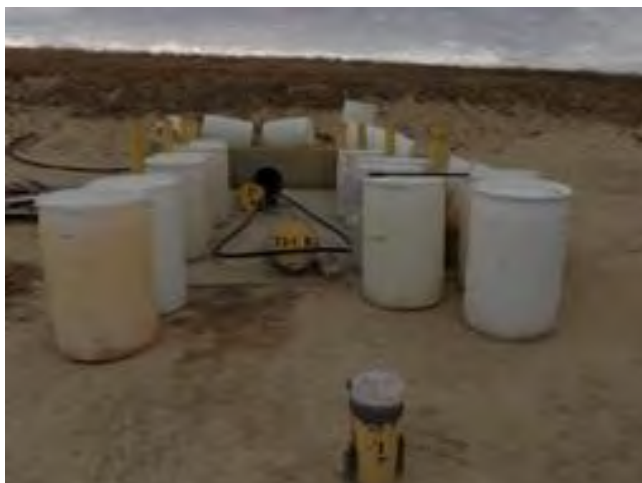
Olympus Stylus 8000, Photo #91; View of the leachate collection system at WMU 33 Cell #1. There are four full and one partially-full 55-gallon containers of F039 leachate in the less-than-90-day storage area.
