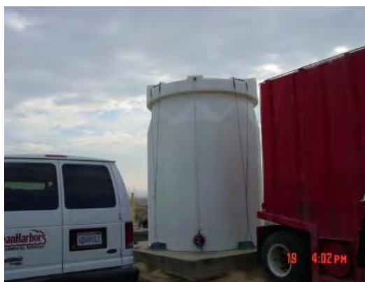
Sony DSC-S75, Photo #11; View of a 5,000-gallon, white plastic, leachate collection tank at WMU 35 Cell #3, facing west.
