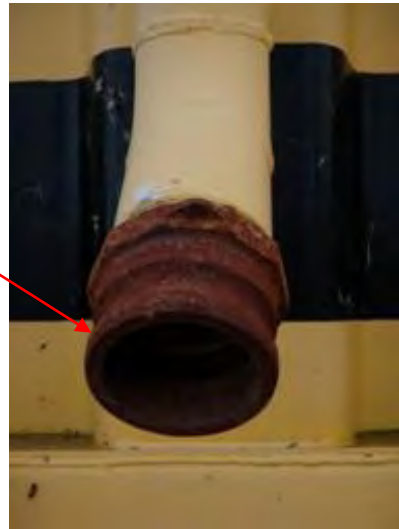
Olympus Stylus 8000, Photo #99; View of the open pumping port at the rear of the leachate collection frac tank (Tank 80) at WMU 35, Cell #1.
