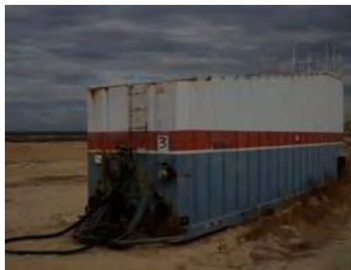
Olympus Stylus 8000, Photo #73; View of the leachate collection frac tank (Frac Tank 3) at WMU 28.
