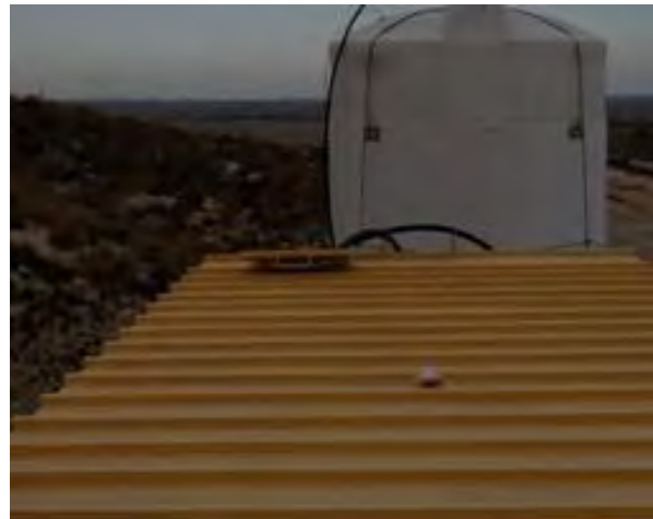
Olympus Stylus 8000, Photo #98; View of the leachate collection frac tank (Tank 80) at WMU 35, Cell #1, shown in Photo 96. Note the top of the container is open.
