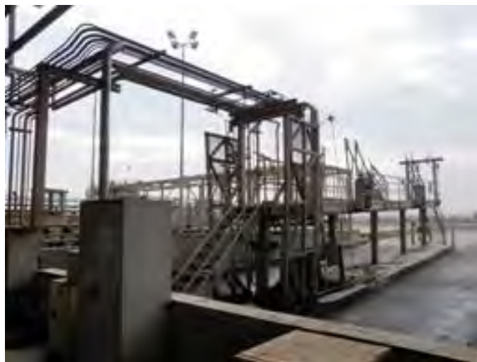
Olympus Stylus 8000, Photo #4; View of the truck wash area at the STU.
