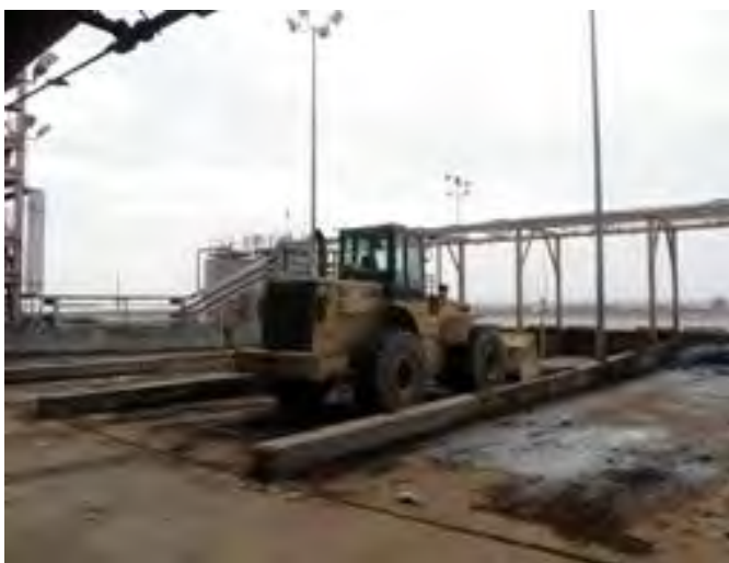
Olympus Stylus 8000, Photo #5; View of the bulk unloading bays at the STU, facing southeast.
