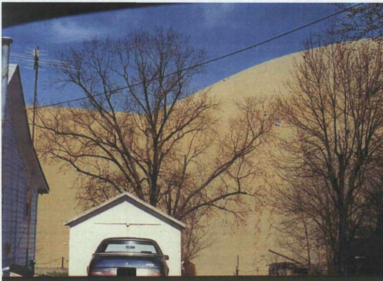
Figure 2. National Pile Before Remediation
