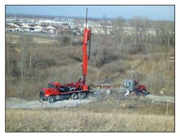
Drilling and core sampling to locate an isolation barrier between West Lake Landfill and Bridgeton Landfill is going on for the next several weeks. (U.S. EPA photo)
