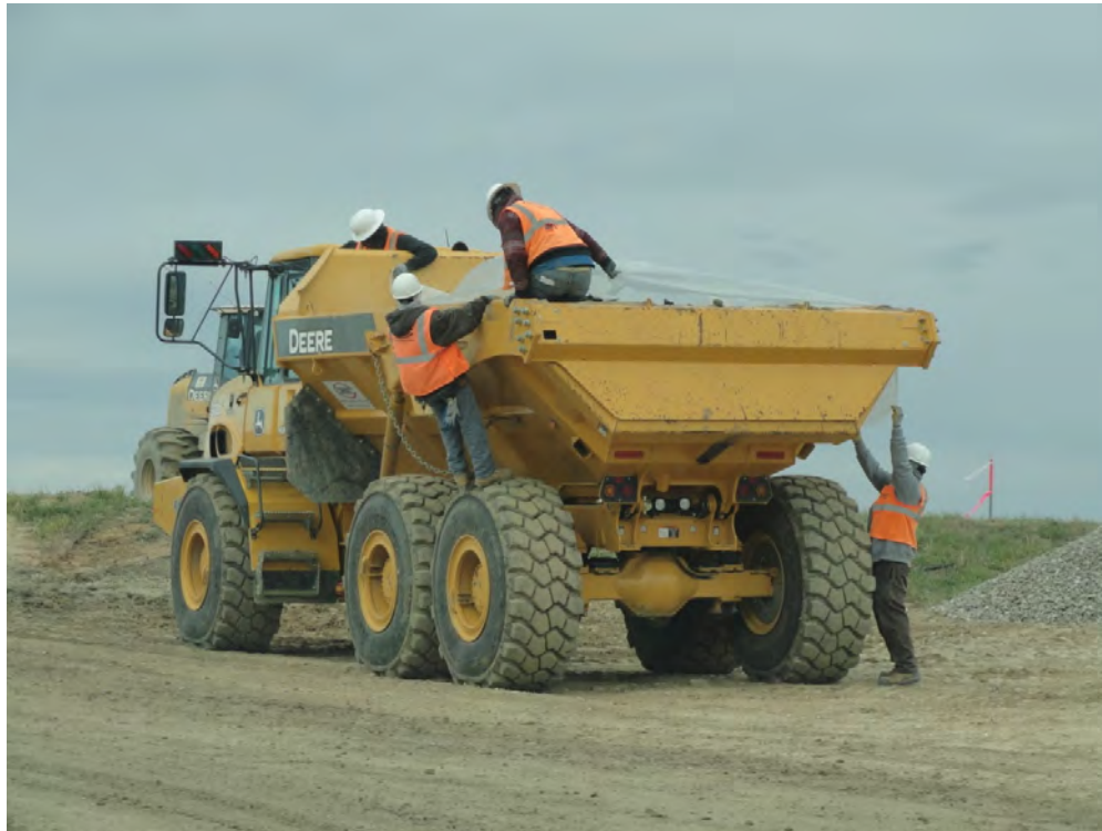
Photo 15: View of Trash being covered before Hauling to Transfer Station.
