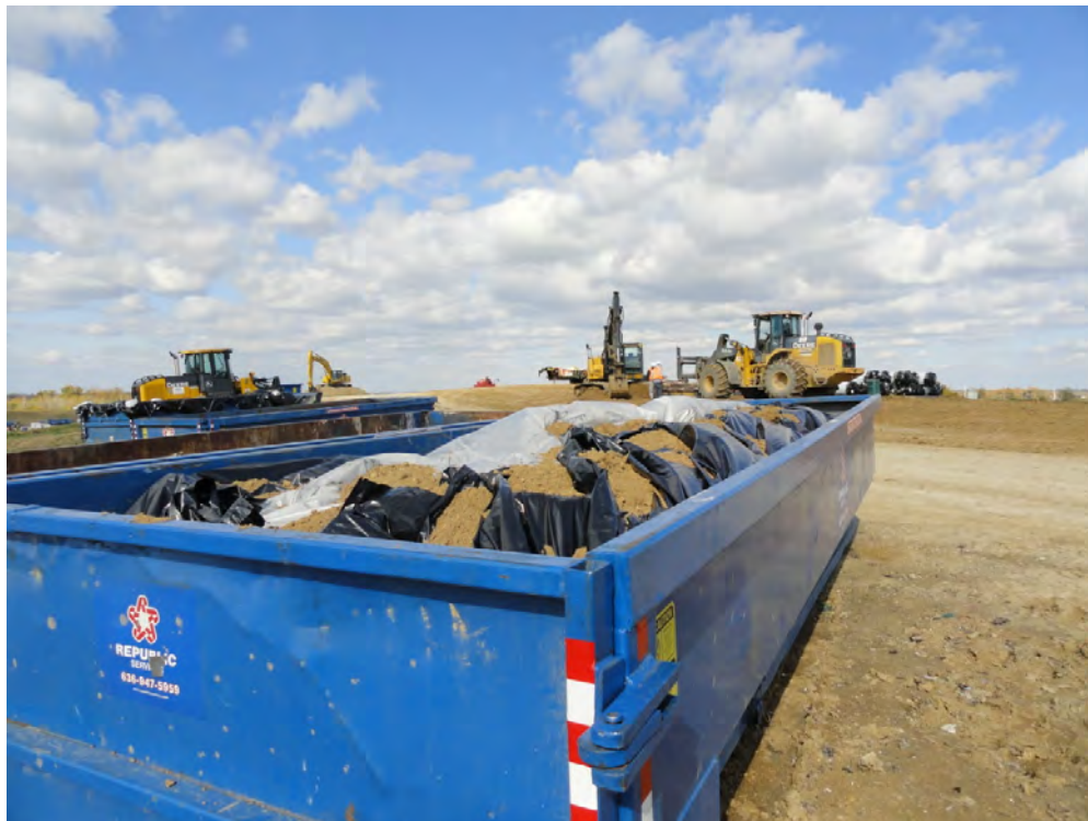
Photo 11: View of Covered Dumpster Box at End of Work Day.
