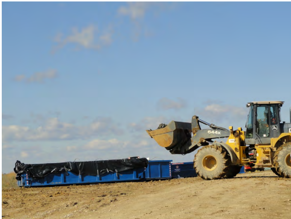
Photo 5: View of Trash being Hauled to Dumpster Box.
