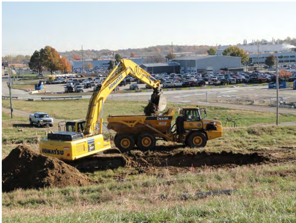
Photo 17: View of Trash being Loaded into Dump truck during Perimeter Sump Installation.
