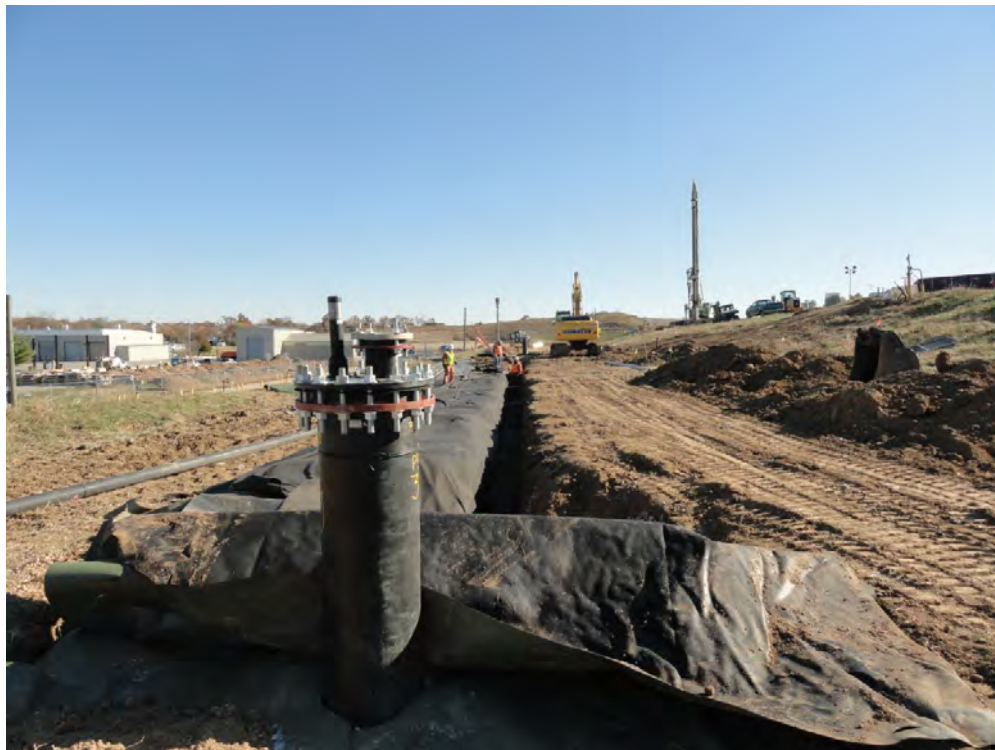
Photo 19: View of Perimeter Sump and Toe Drain Installed.
