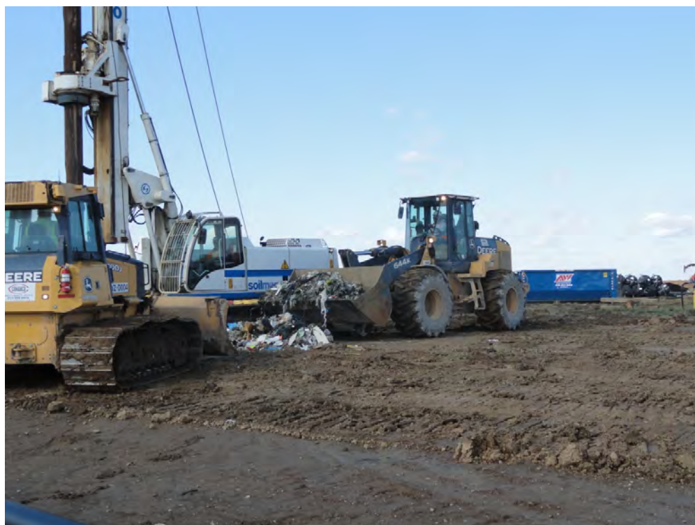
Photo 4: View of Trash Removal during Gas Extraction Well Installation.
