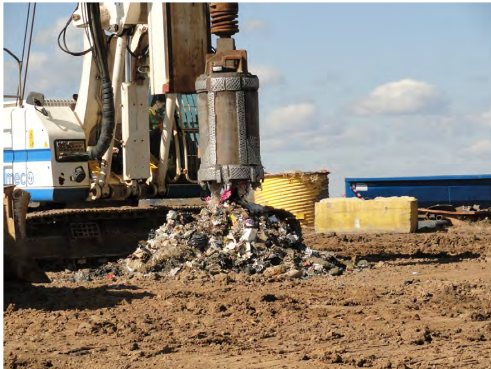
Photo 3: View of Trash from Drill Bit during Gas Extraction Well Installation.
