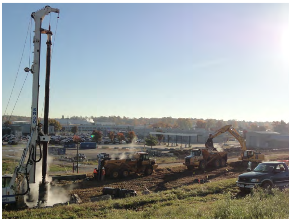
Photo 18: View of Gas Extraction Well and Perimeter Sump Installation.
