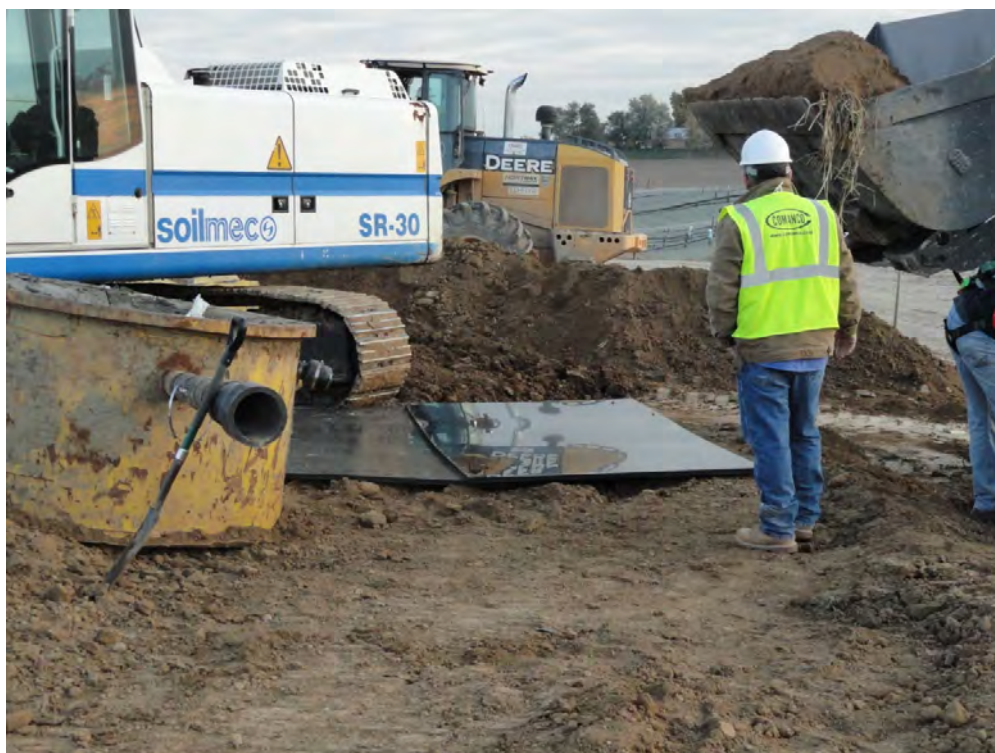
Photo 10: View of Partially Finished Gas Extraction Well Hole being Covered at End of Work Day.
