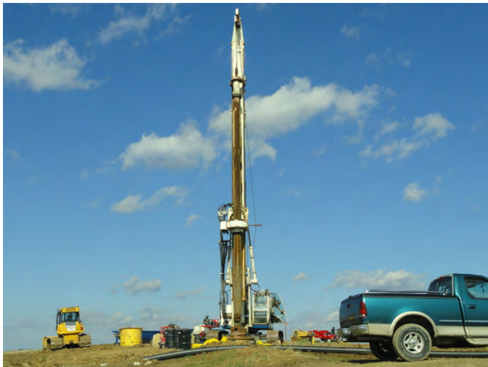
Photo 2: View of Gas Extraction Well Drill Rig.
