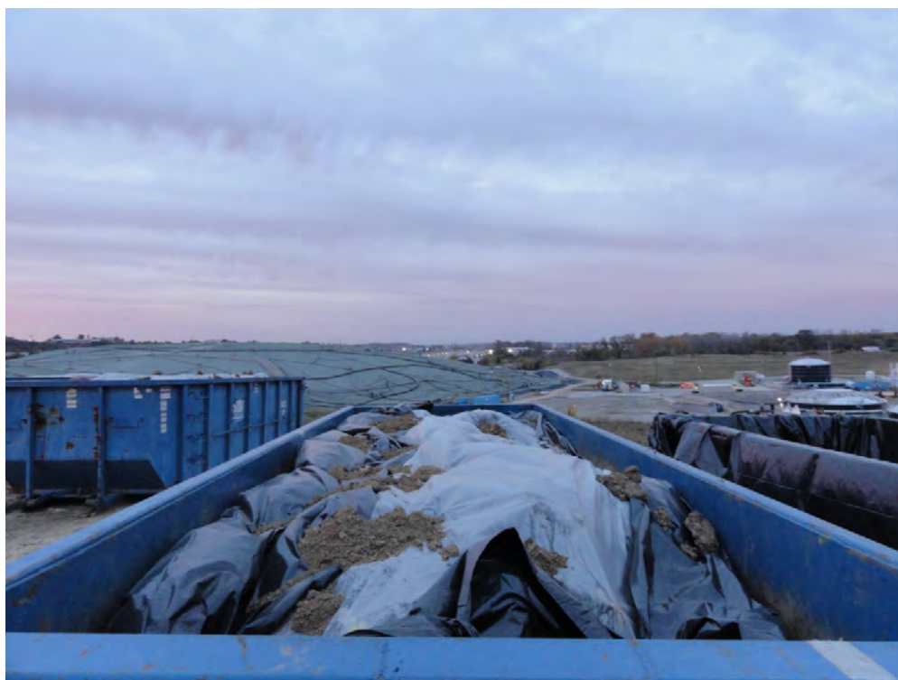
Photo 12: View of Covered Dumpster Box at Beginning of Work Day.
