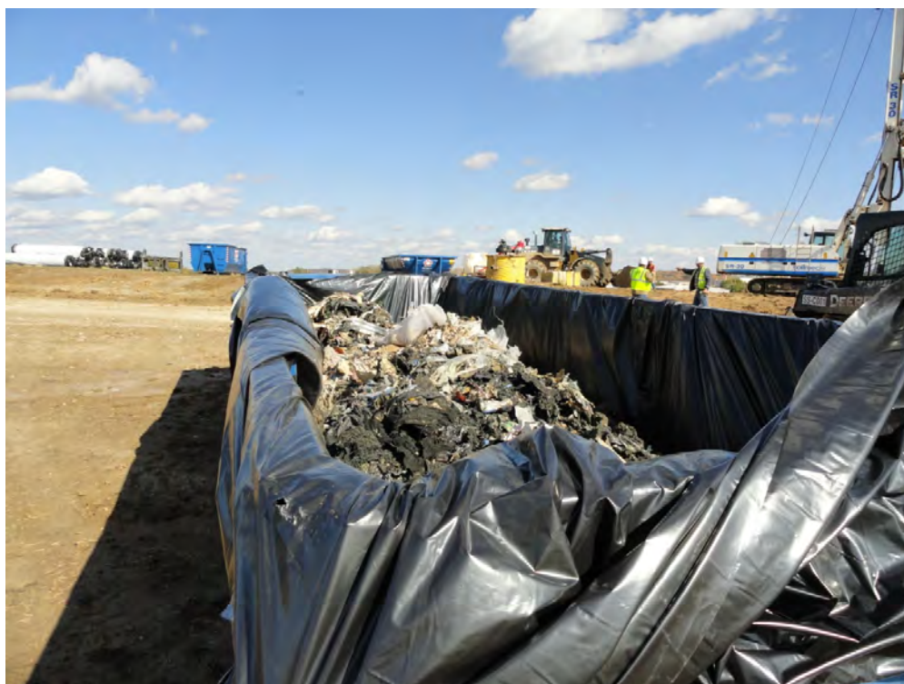
Photo 6: View of Trash in Dumpster Box.
