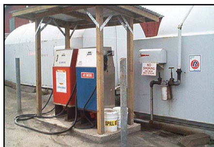
Figure 8. Spill kits should be maintained in areas with spill potential, such as fueling stations.
