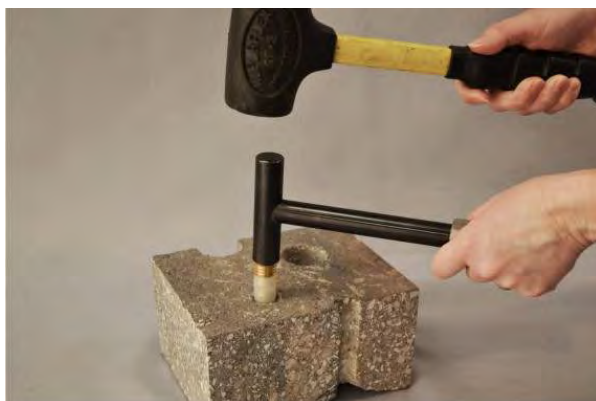
Figure 2. Installing the Vapor Pin™.
