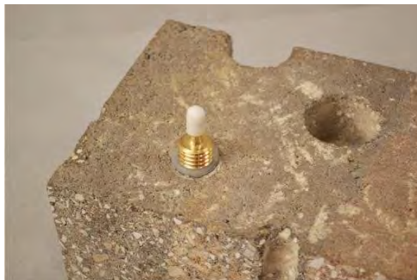
Figure 4. Installed Vapor Pin™.
