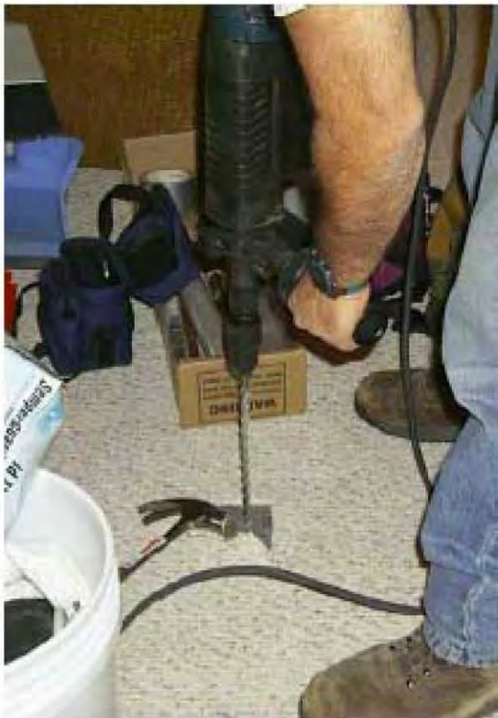
Figure 1. Drilling through a slab
