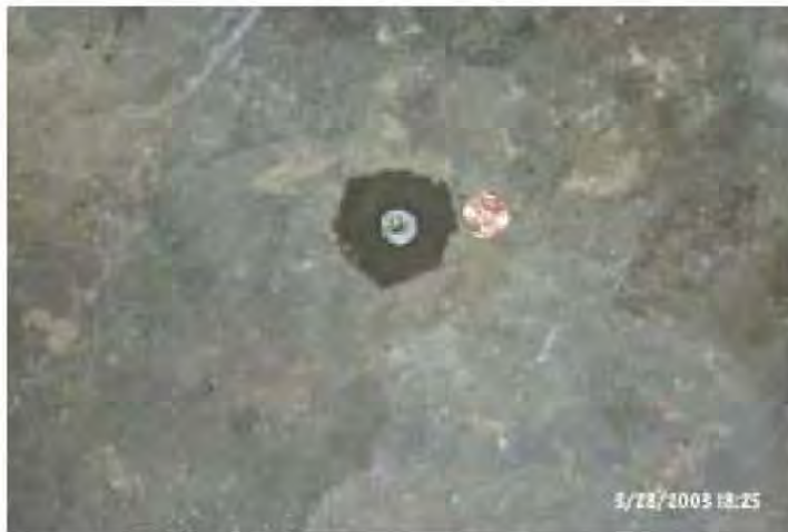
Figure 5. Completed vapor probe installation
