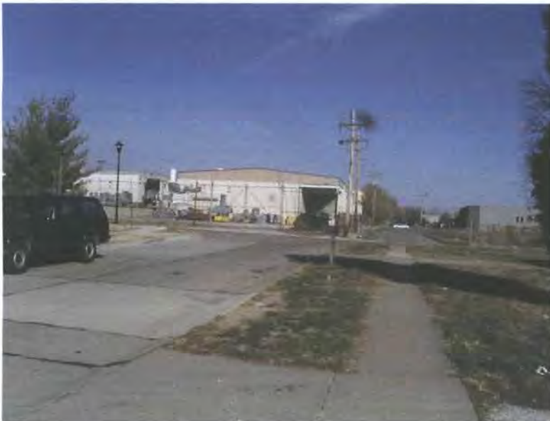
Photo 8. Chicago Heights Blvd VOC Plume site, Overland, MO. Photo taken on December 1, 1999 by Nancy Priddy, Superfund, DNR. View of industry north of site. Taken from Elmridge Place looking north.
