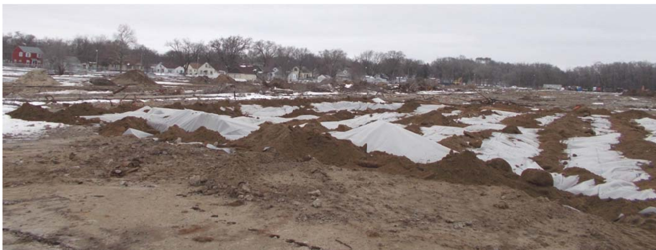
View looking northwest across Area 6-1 with plastic cover. Plastic covered mounds on southern
