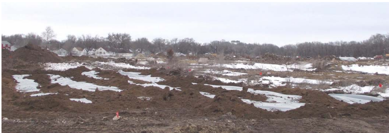
View looking north across Area 5-12 with plastic cover. Red flags mark east and south sides Area 5-12.
