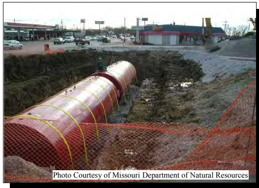
INSTALLATION OF AN UNDERGROUND STORAGE TANK
