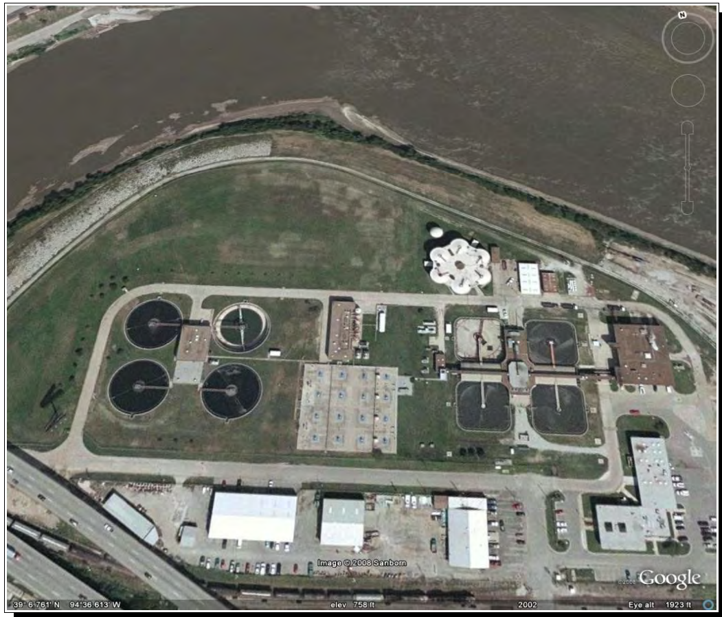
PUBLICLY OWNED TREATMENT WORKS FACILITY
