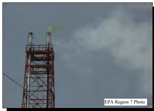
PROCESS STREAMS CONTAINING METHANOL SHOULD BE VENTED TO A FLARE
