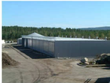
Process modules and biogas reactor
