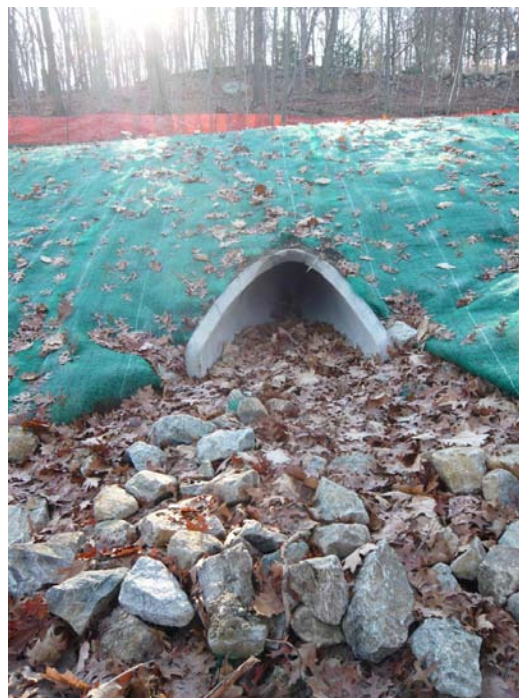
Figure 4.28 Completed drainage culvert with stone outfall protection.
