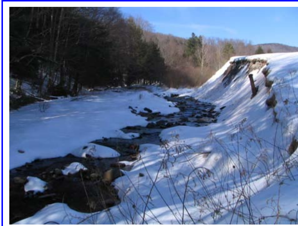
Figure 4.21a Horton Brook before floodplain restoration.
