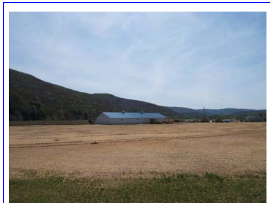
Figure 3.2. Hamden leach field and sand filter building.
