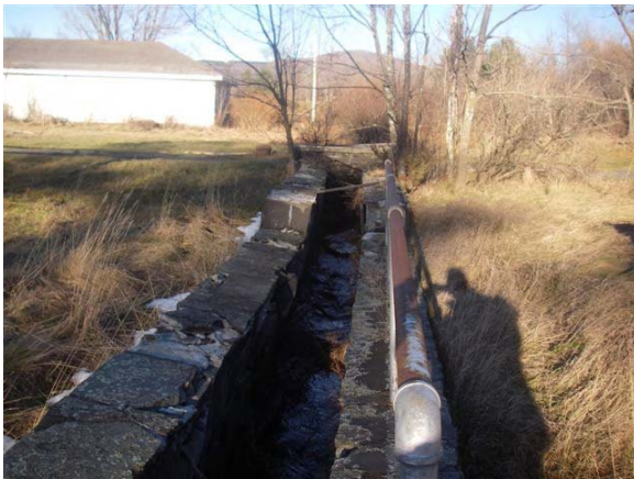
Figure 4.18a Before Sugar Maples stream restoration.
