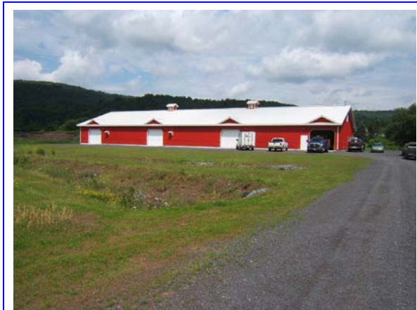
Figure 3.1. Bloomville sand filter building.
