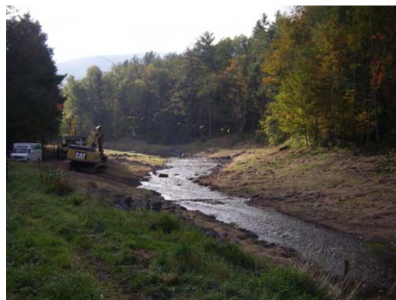
Figure 4.17c Long Road after restoration.
