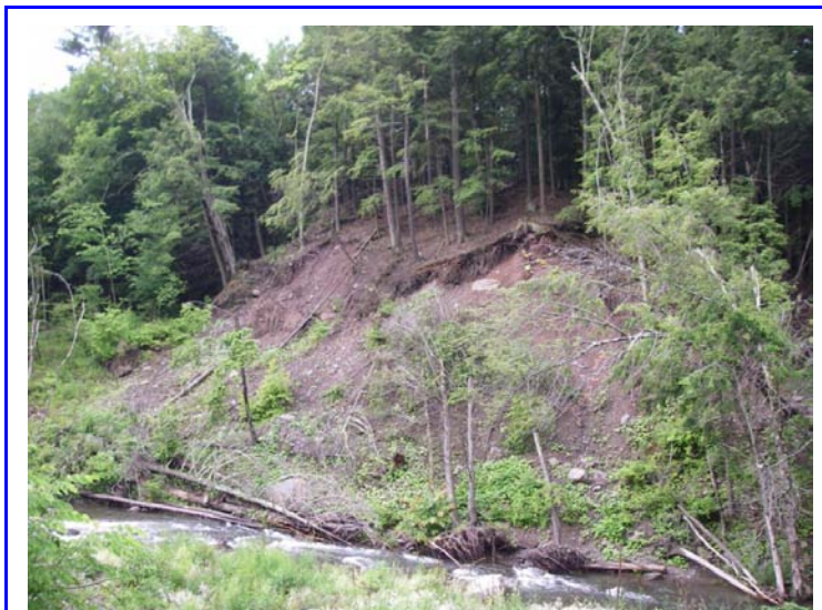
Figure 4.18a Long Road before restoration.
