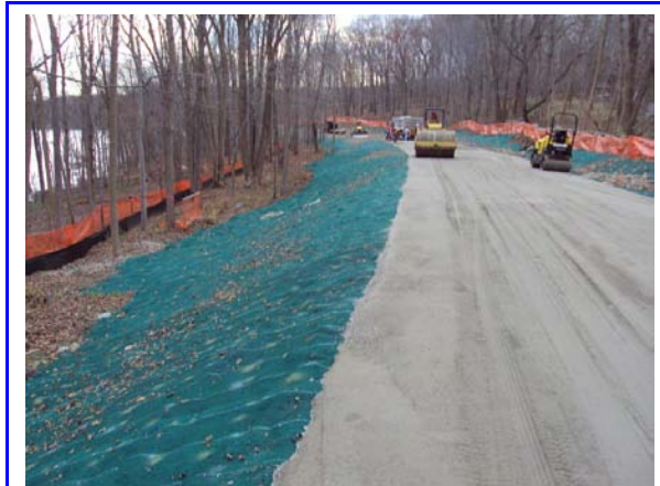
Figure 4.27 Completed erosion protection on slope.
