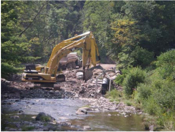
Figure 4.17b Long Road during restoration.
