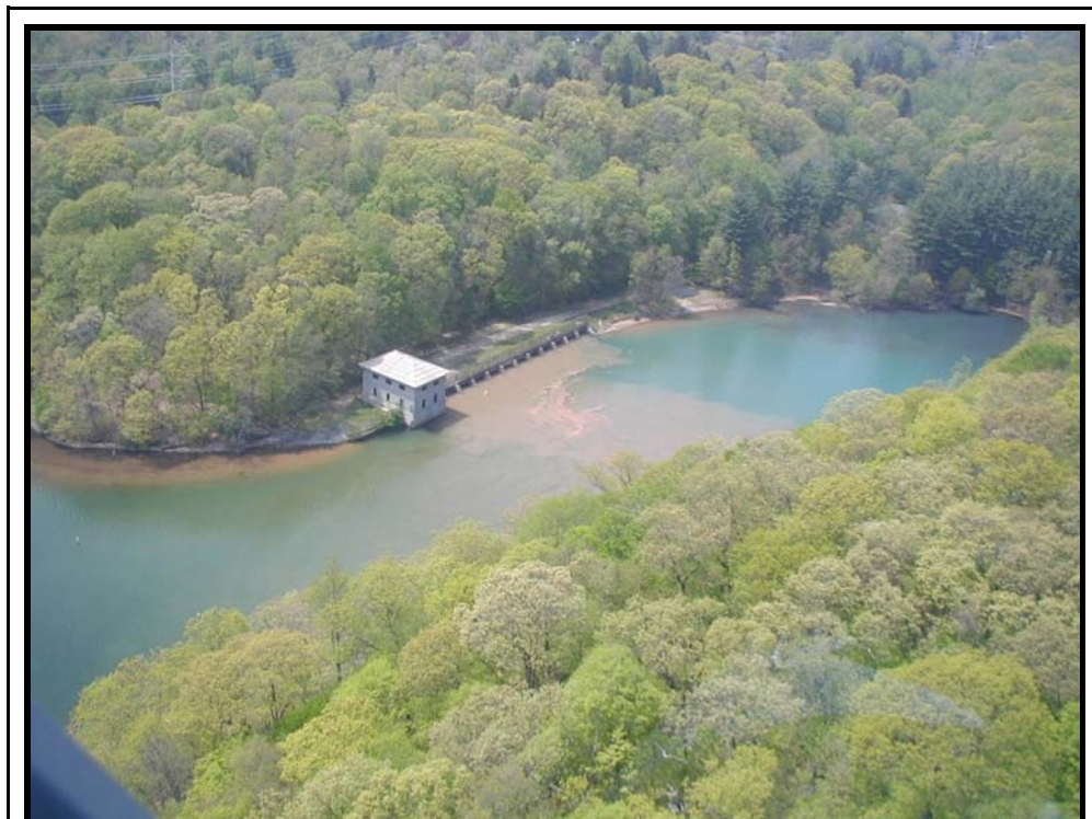
Figure 1.7 Photograph of the Catskill Inflow Chamber Cove on Kensico Reservoir taken in May 2005 during alum treatment (looking approximately northwest).
