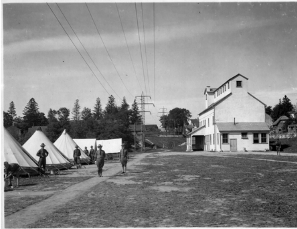
Figure 1.6 This picture of New York City's Board of Water Supply coagulating plant, taken September 19, 1917, indicates that turbidity was an anticipated water quality concern.
