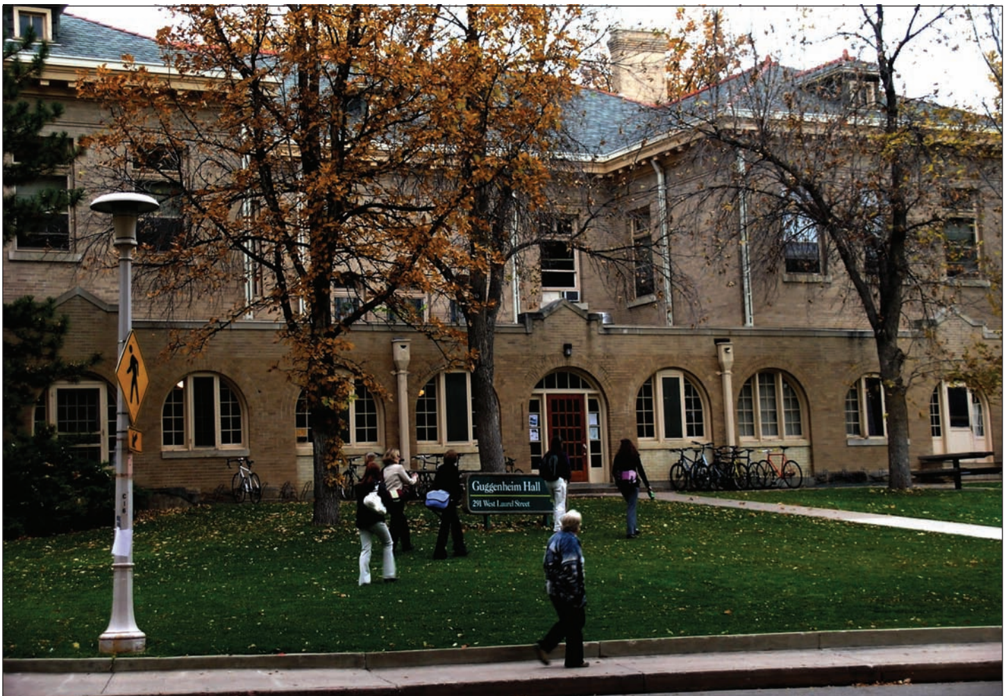
Guggenheim's second floor classrooms at Colorado State University obtained LEED Silver Certification.
