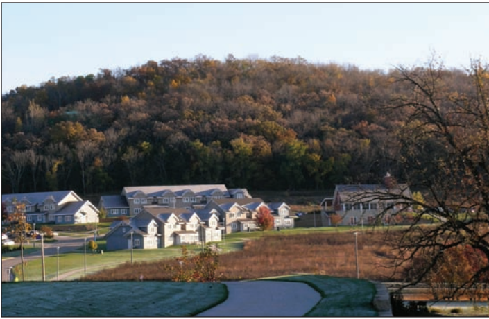
Baker Village student housing at Luther College includes geothermal heating and cooling.
