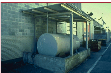
7 - Covered AST with secondary containment (above)
