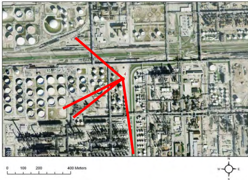
Figure 3-5. Proposed Dial Location 4: Shell Deer Park: OP2 and OP3 elevated flares (OP2ELFLA & OP3ELFLA), OP3 ground flare (OP3GRFLA) and certain tanks north of the olefins units. This location may also be good for olefins units cooling towers and process unit fugitives
