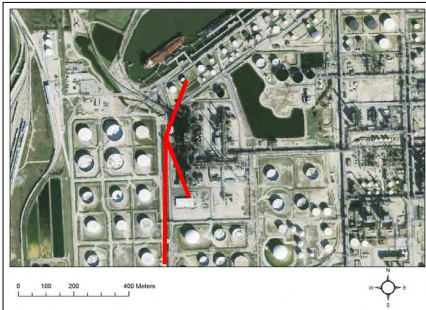
Figure 3-7. Proposed Dial Location 6: Coker units and tanks generally east of coker units
