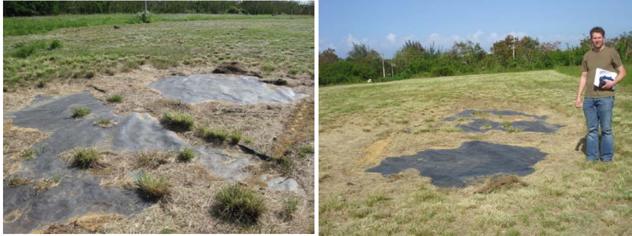
Figure 6. Views of the exposed impermeable plastic liner of the Cataño Landfill cap
