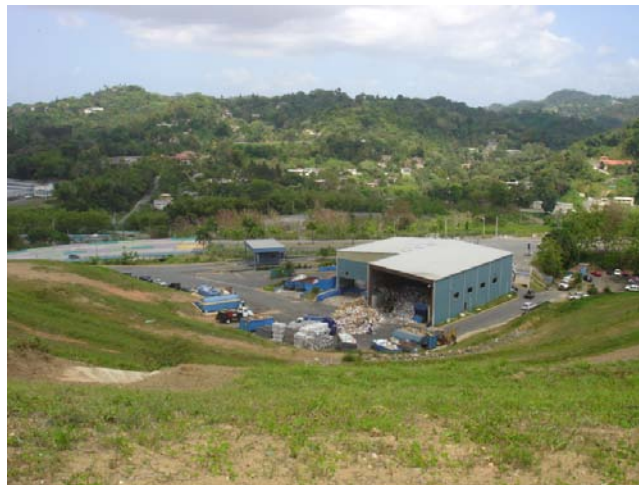
Figure 13. Guaynabo Landfill recycling center
