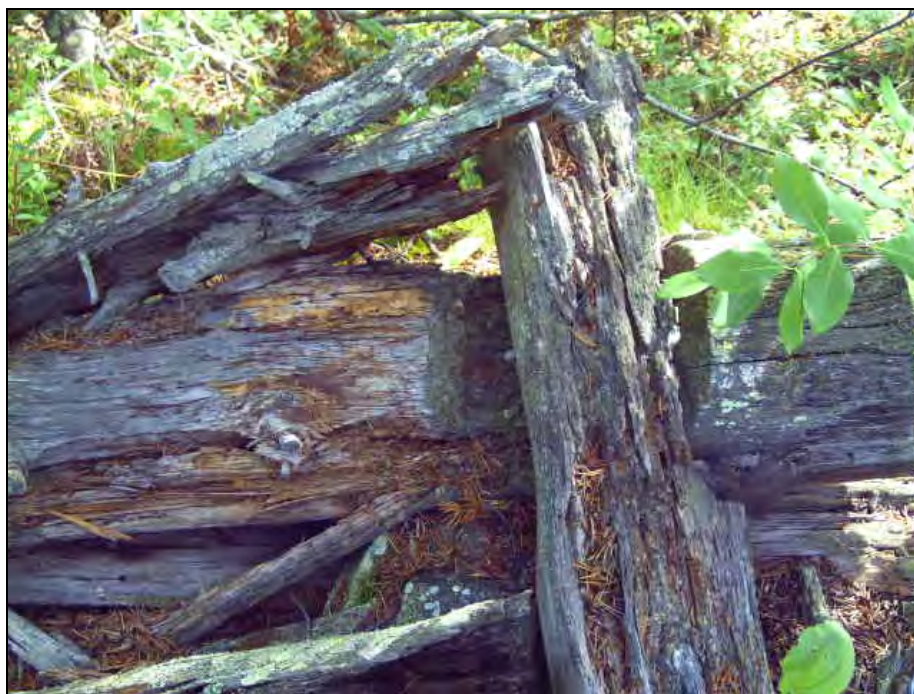
Close-up view of construction of Structure #1 at 20Mq229.
