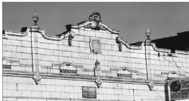
Figure 30. Ornate parapet of a building on the 1700 block of Broadway.
