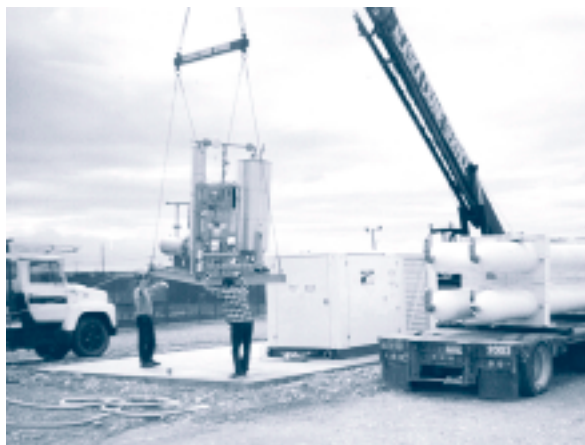
Figure 10 Construction of the CNG fueling station at Elmendorf AFB.
