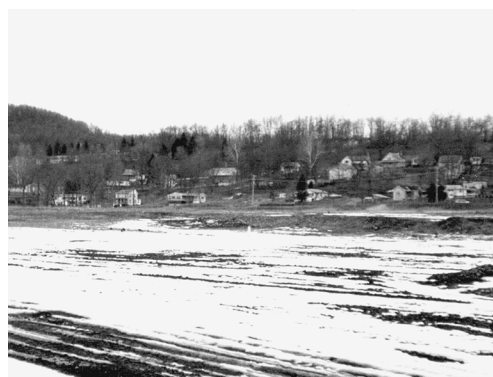
Fairmont Coke Works — 2/10/2000 — By the winter, all demolition work is complete. This view looks across the snowcovered site, now leveled for future redevelopment.
