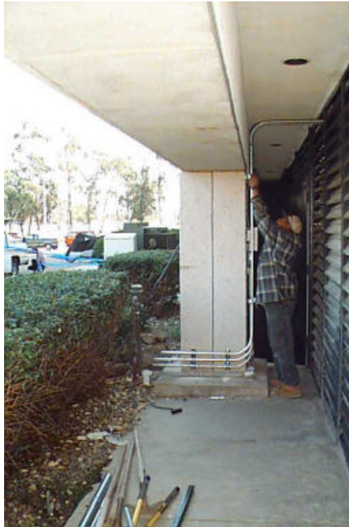
Above ground conduit providing power to each charging station.
