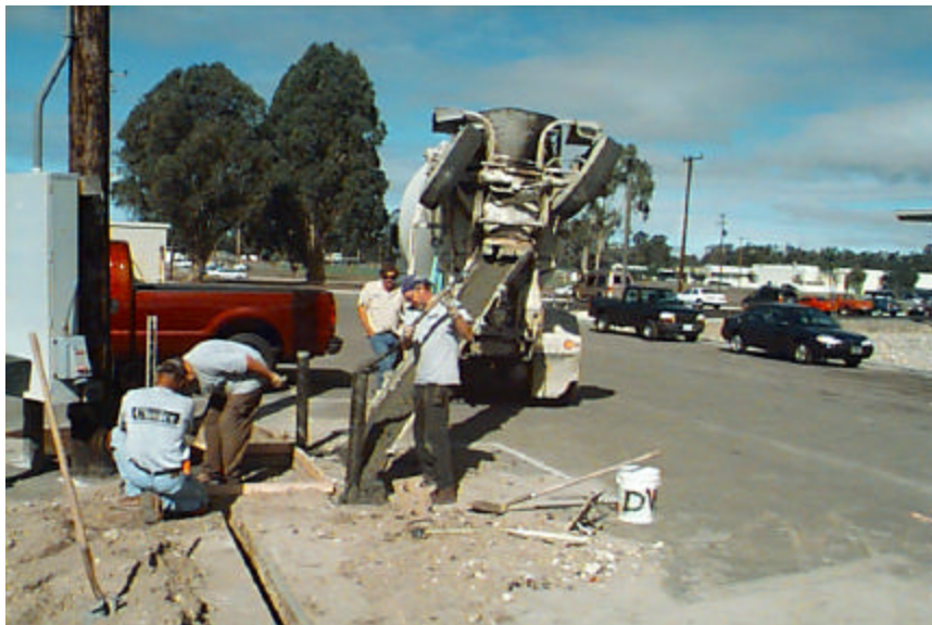
Concrete footers are poured to support the charging stations, a small step-down transformer and safety ballards around the installation.
