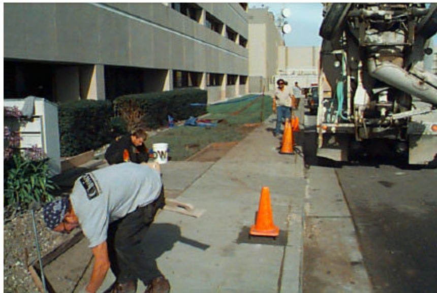
Concrete footers were poured for each pedestal mounted charging station and sidewalk widths were increased to meet ADA requirements for ease of handicap access around charging stations.
