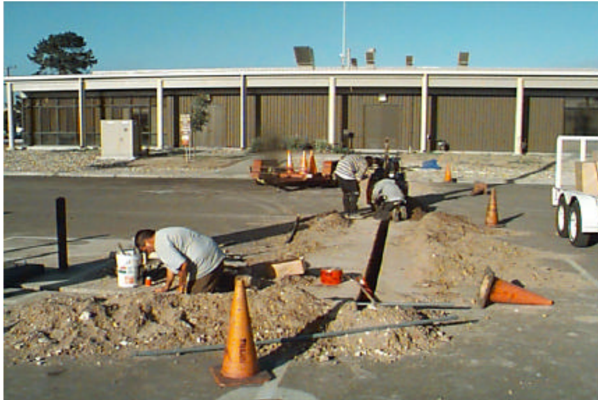
Under ground conduit providing power to each charging station.
