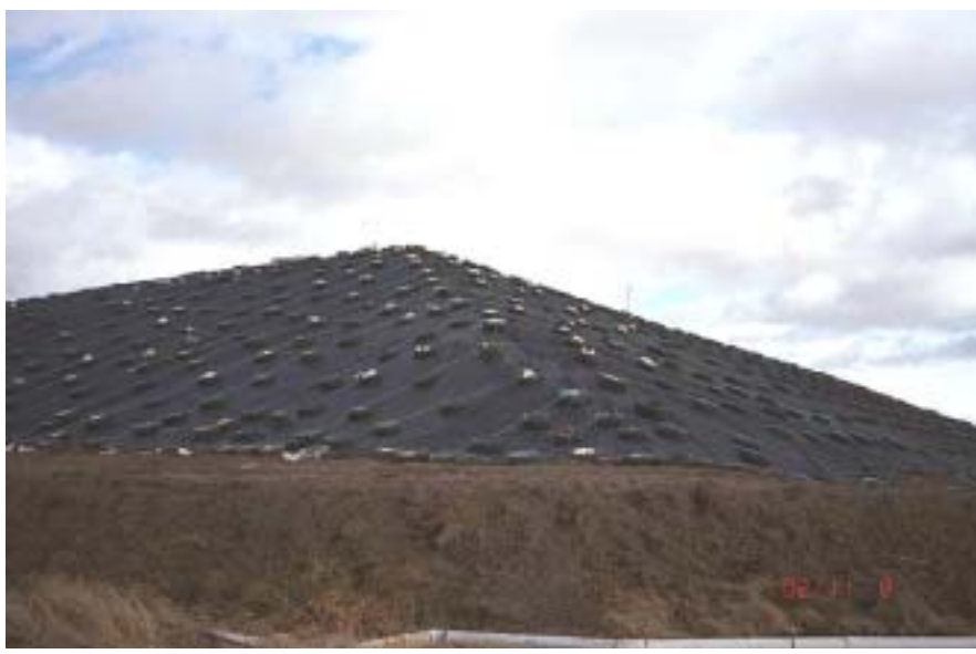
Image 4-4. West-side anaerobic cell surface liner.
