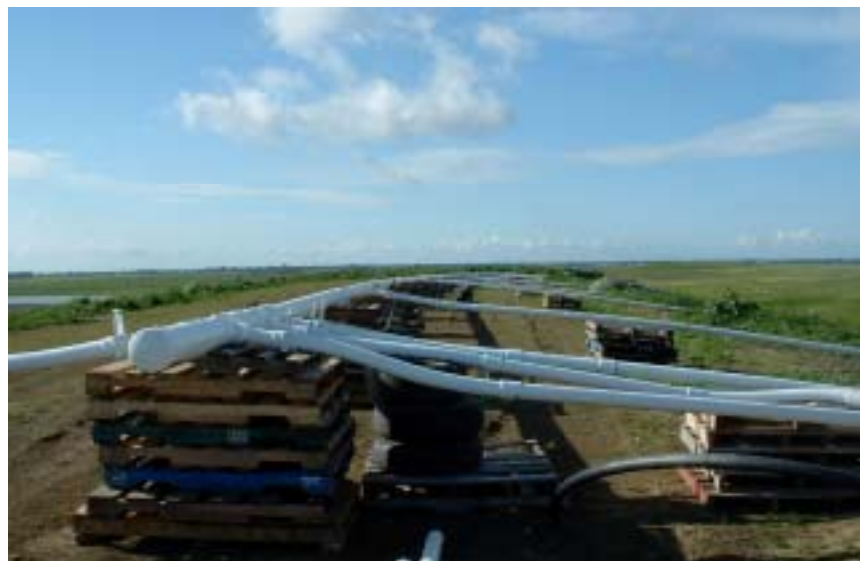
Image 4-3. LFG collection laterals connected to the main header line located on top the cell.
