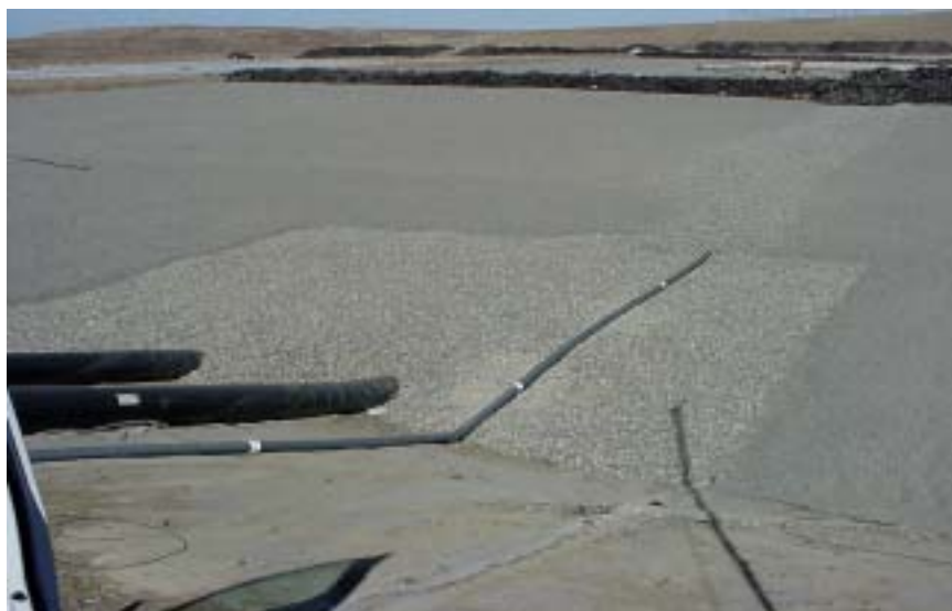
Image 3-5. Gravel drainage layer and leachate collection sump
