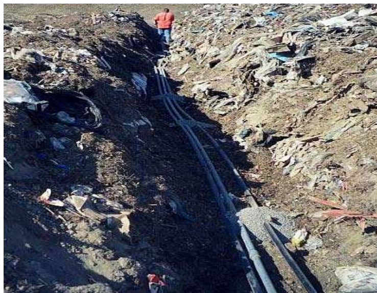
Image 5-2. Leachate injection laterals in trench
