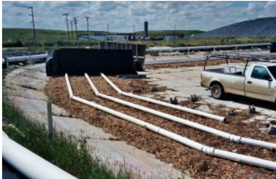
Image 5-7. Construction of the biofilter
