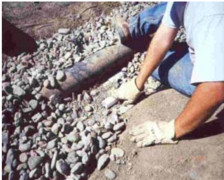
Image 6-2. Pressure tubes installed in LCRS trench
