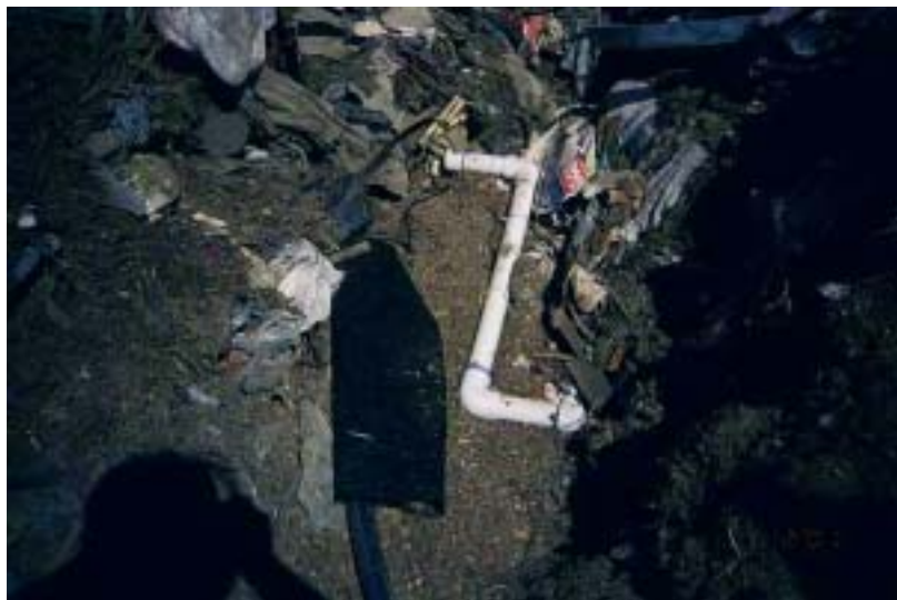
Image 3-4. Moisture, temperature , and tube installation
