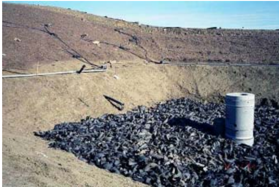
Image 5-4. Aerobic sump installed and ready for backfill
