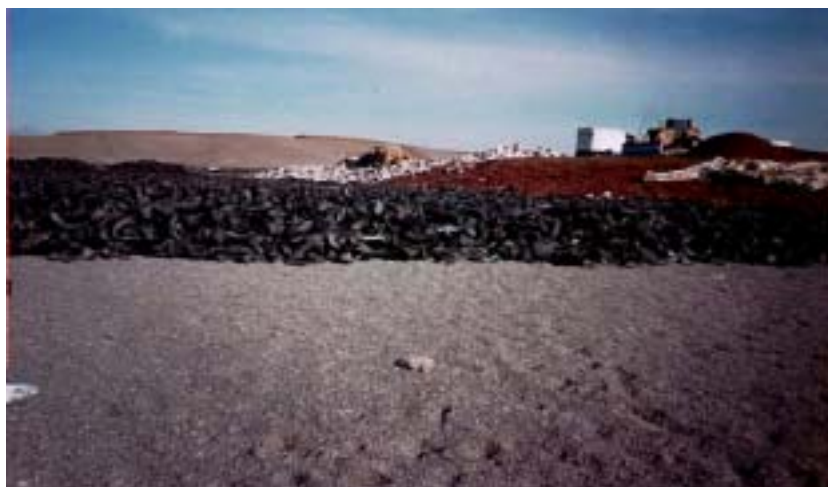
Image 6-1. Shredded tire operations layer
