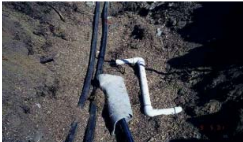
Image 5-3. Moisture, temperature, and tube installation
