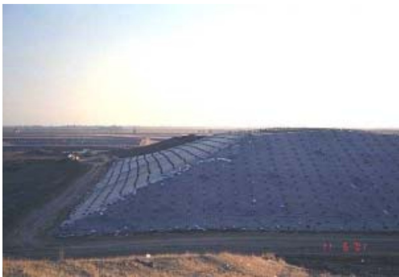
Image 3-3. Northeast anaerobic surface liner
