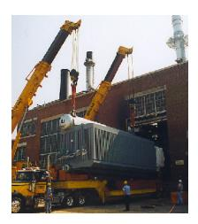
Gas boiler being positioned for installation in the powerhouse
