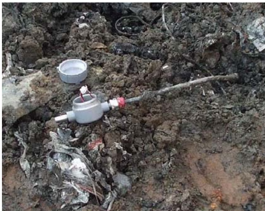
Figure 2-9 Installation of Thermocouples in Cell 6
