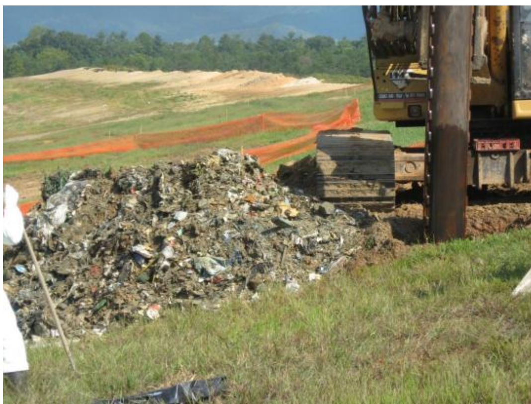
Figure 5-6 Exhumed Waste from Drilling of Vertical Well 13
