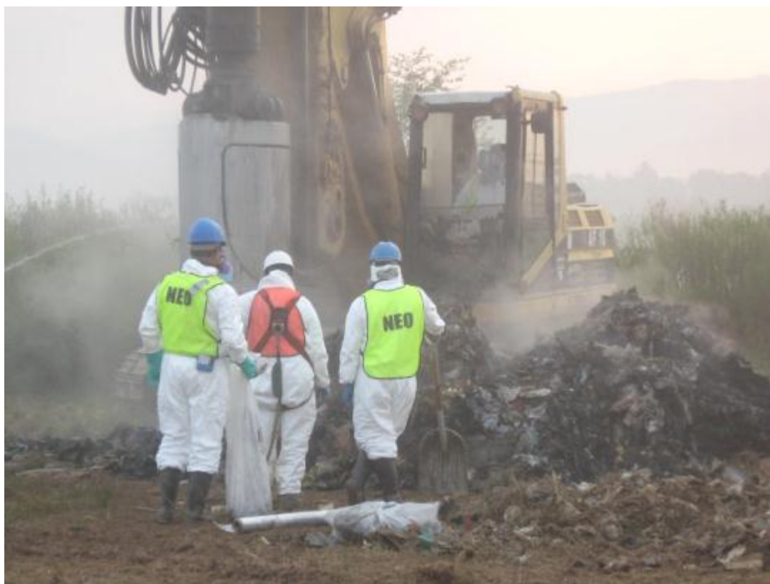
Figure 5-5 Exhumed Waste from Drilling of Vertical Well 24
