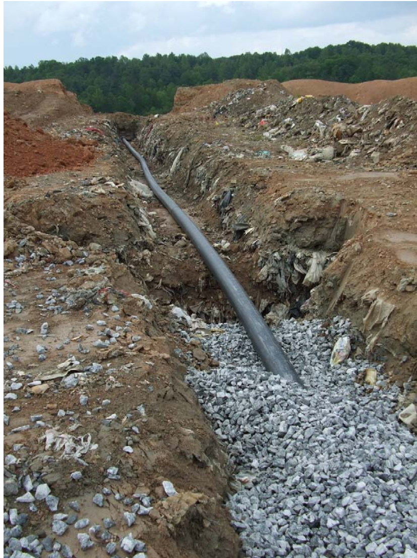
Figure 2-7 Horizontal Injection Trenches in Cell 6
