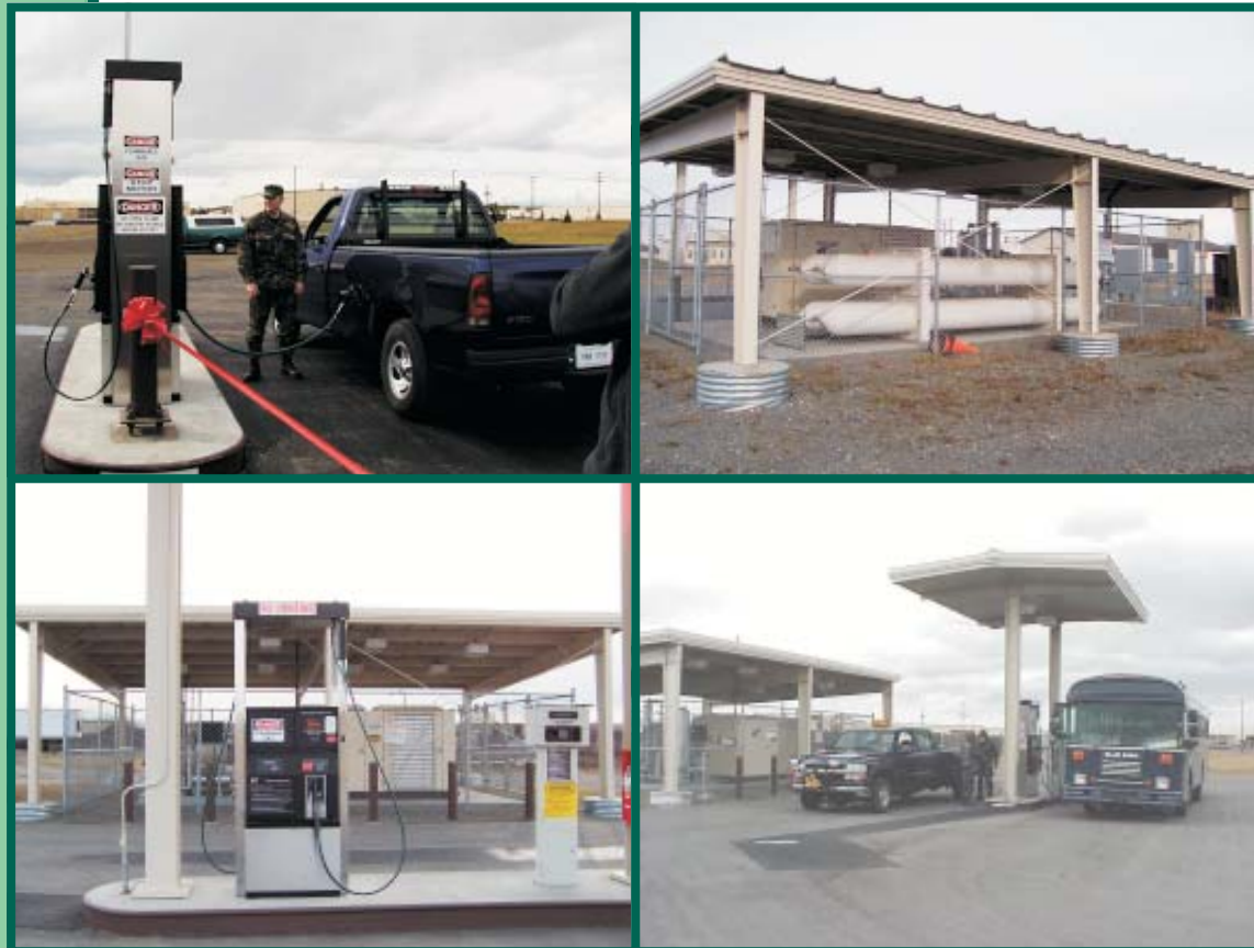
CNG Fueling Station, clockwise from top left: First customer, CNG fueling station dedication ceremony, April 2000; canopies were added in 2002 to enhance usability and maintenance by protecting the gas cylinders and dispenser island; Elmendorf's 44-passenger shuttle bus was converted to a dedicated CNG engine; state-of-the-art fuel dispenser is integrated with a Fuel Master® tracking system, which logs gas usage by vehicle.
