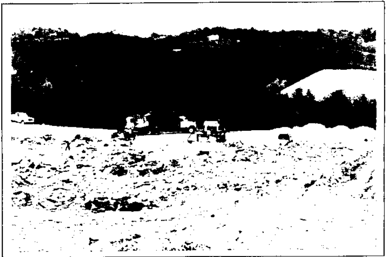
Photograph 14. C&D waste is compacted continuously and covered once per week. C&D diversion saves valuable space in the Subtitle D Landfill.
