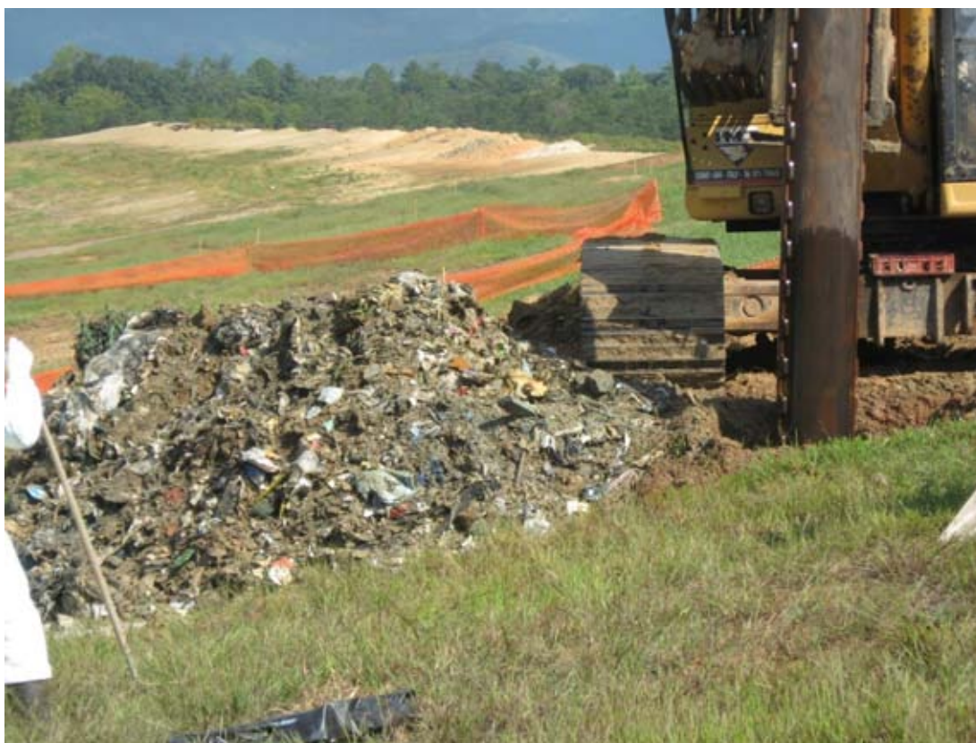
Figure 5-6 Exhumed Waste from Drilling of Vertical Well 13
