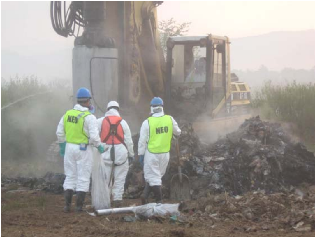
Figure 5-5 Exhumed Waste from Drilling of Vertical Well 24
