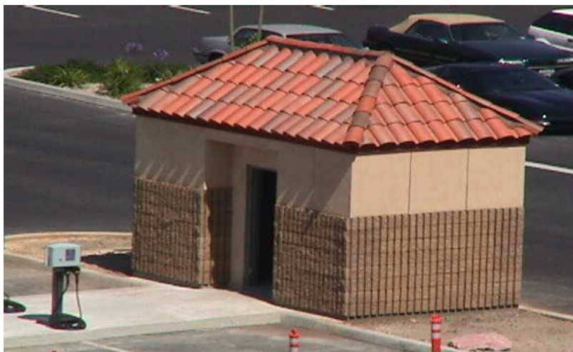
Figure 4 SUVMS Communications Equipment Enclosure
