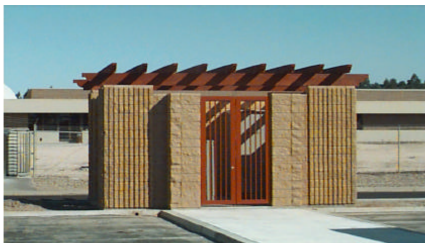
Figure 3 SUVMS Electrical Equipment Enclosure
