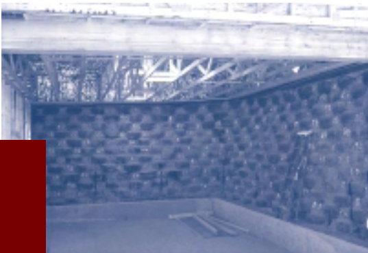
Tires and dirt are used to construct the conference room walls.
