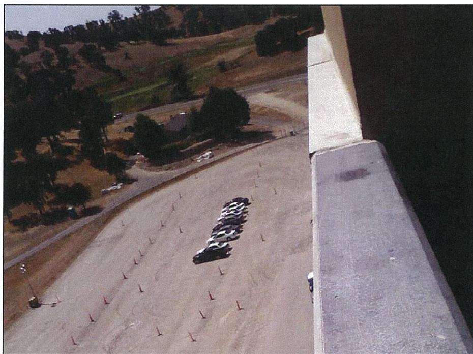
PHOTO 12: Unpaved parking lot at the east end of the parking garage.
