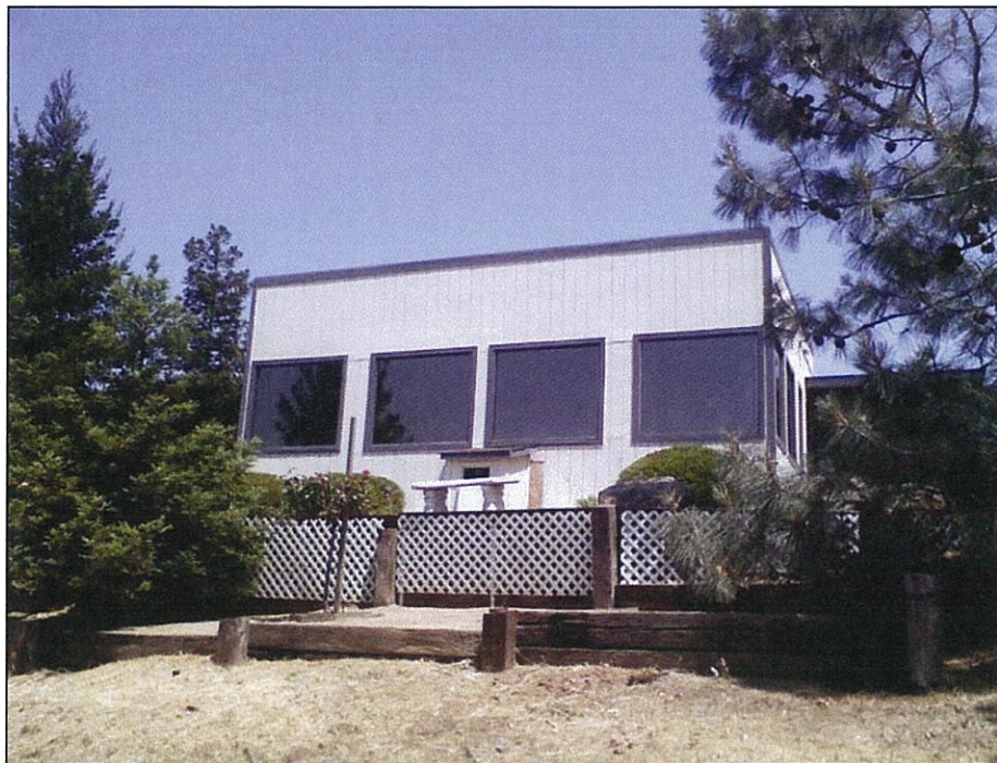
PHOTO 11: South face of the medical building on the upper Rancheria.
