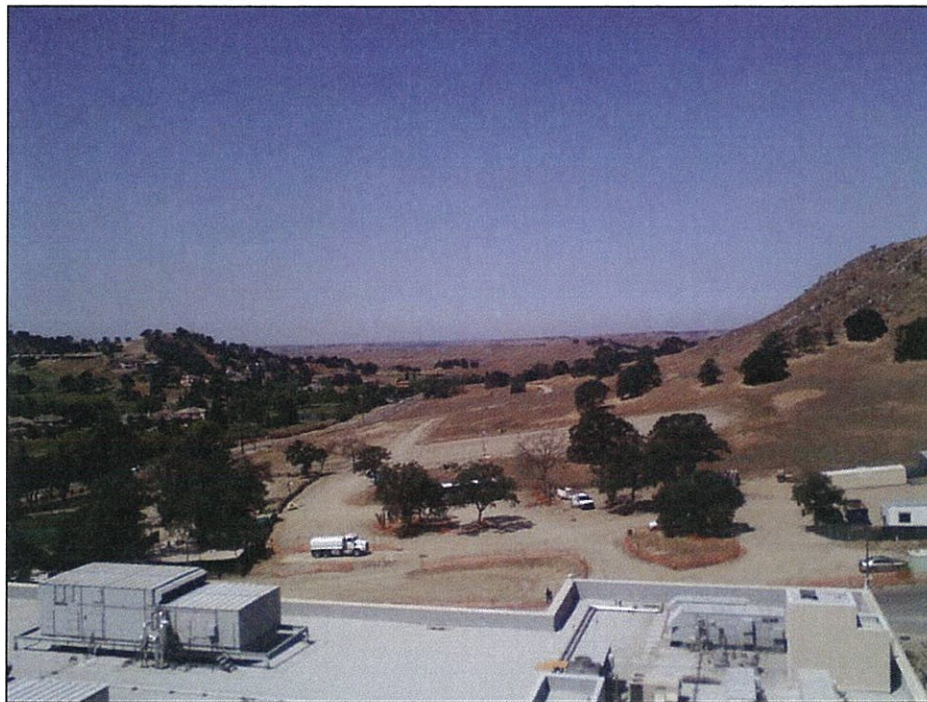
Photo 1: Valley Corridor, view to the west from the parking garage.
