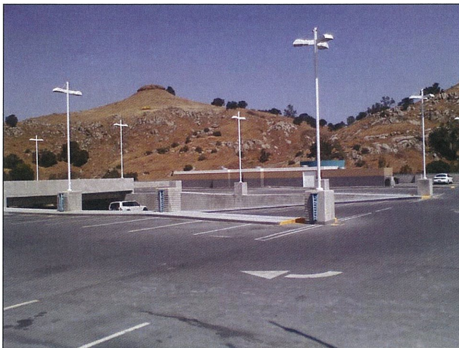
PHOTO 5: Top floor of the casino parking garage, garage and kitchen exhaust, view to the north from the communications building
