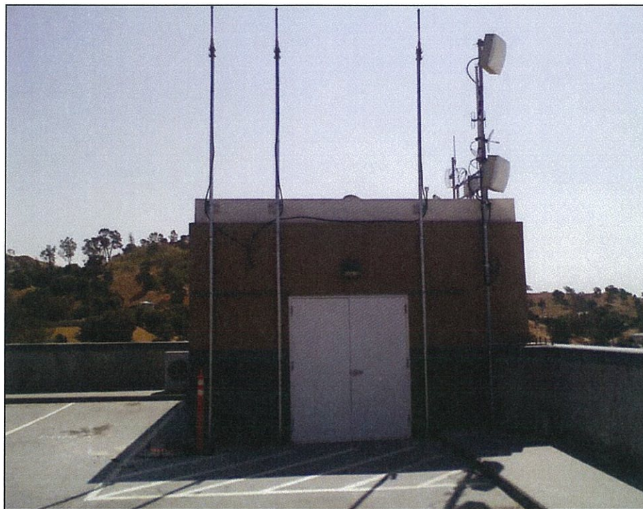
PHOTO 9: Communication building on the southeast corner of the casino parking garage.
