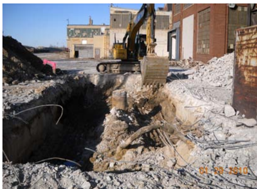
Exposing underground storage tanks to address contaminated soils at the former Tower Automotive/A.O. Smith site
