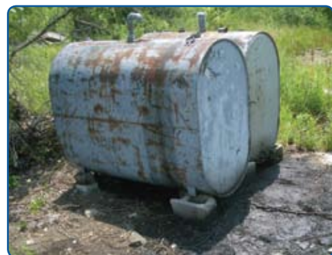
Release of fluids from above ground storage tanks in poor condition with no label.
