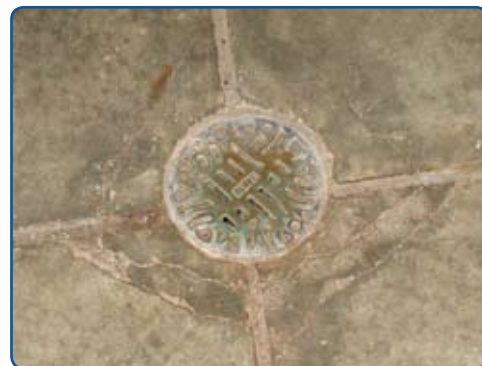
Filled in floor drain.
