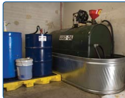
Used oil storage tank in secondary containment.
