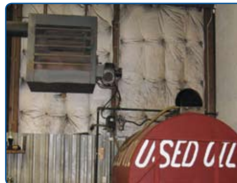
Space heater with labeled used oil storage tank.
