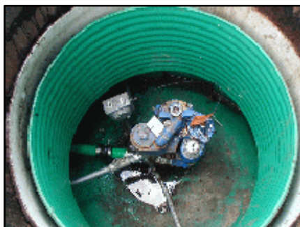
Sample Flexible Piping in a Sump
