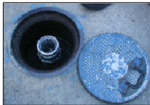
Sample Spill Protection
