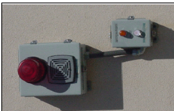
Sample Overfill Alarm
