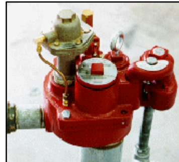
Sample STP Head with LLD
