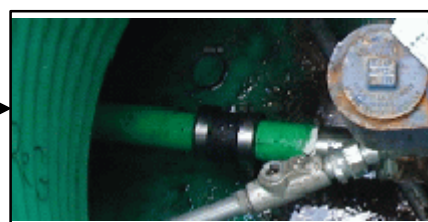
Close-up of Flexible Piping in a Sump
