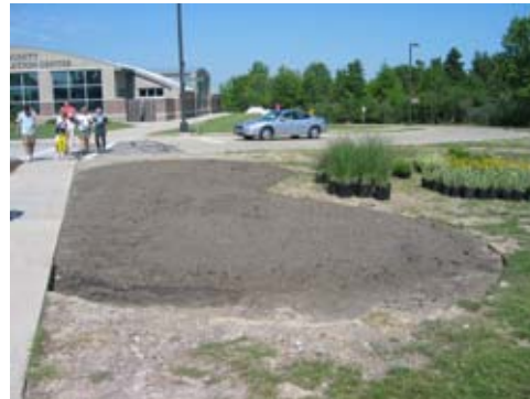
Figure 2. The site after excavation. Gravel and soil mix layers in place.
