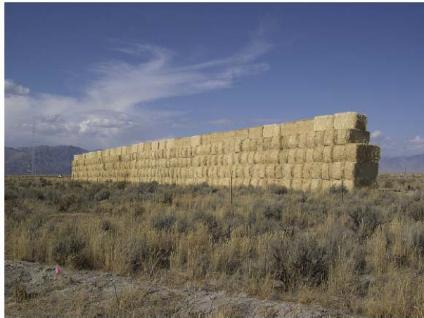
Fig. 1. Mock straw bale sound barrier, 6 m high and 90 m long.
