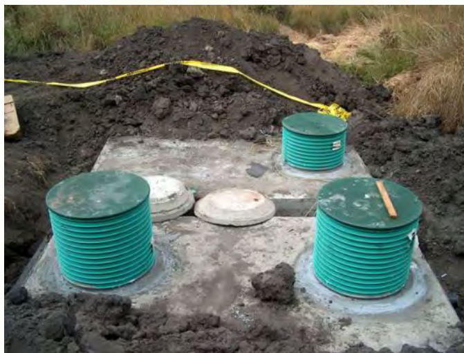
Installation of an advanced treatment system.
