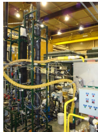
Membrane Assisted Vapor Stripping unit at EPA's Test & Evaluation Facility.
