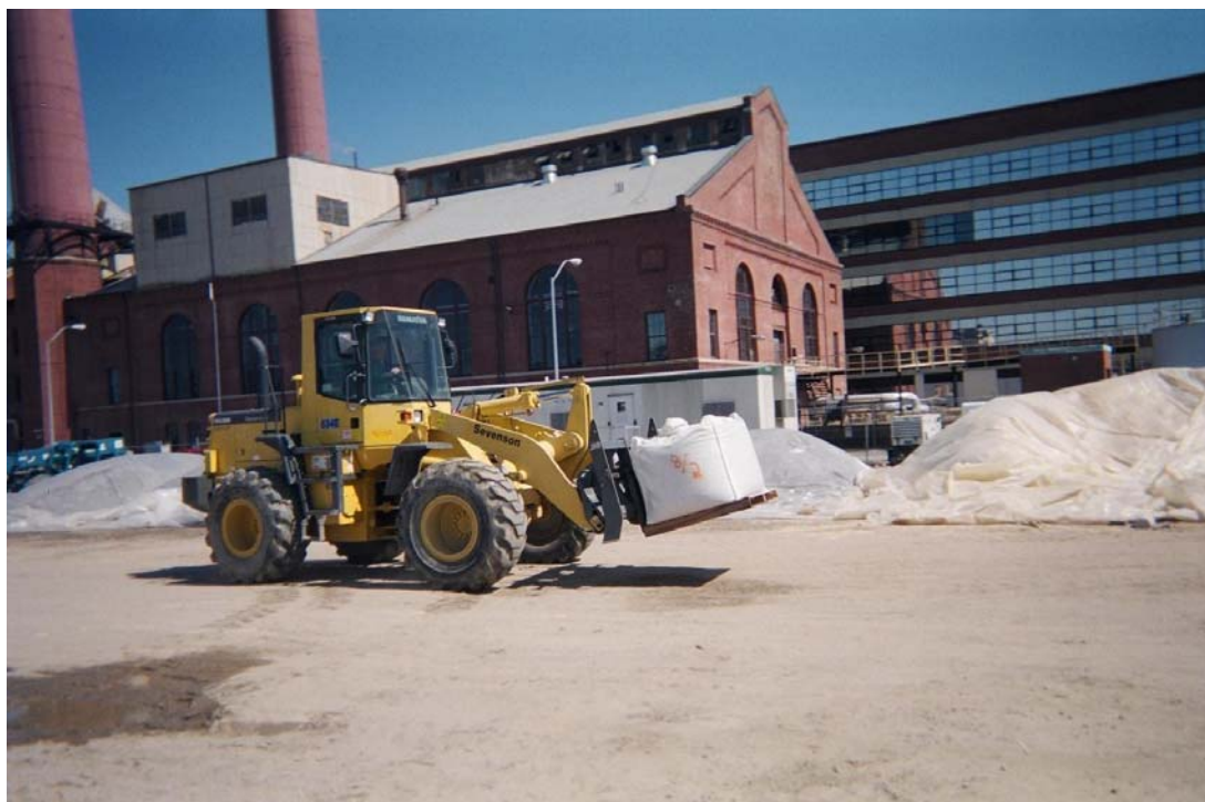
Figure 3-5. AquaBlok® in 2-Ton SuperSack at Staging Area
