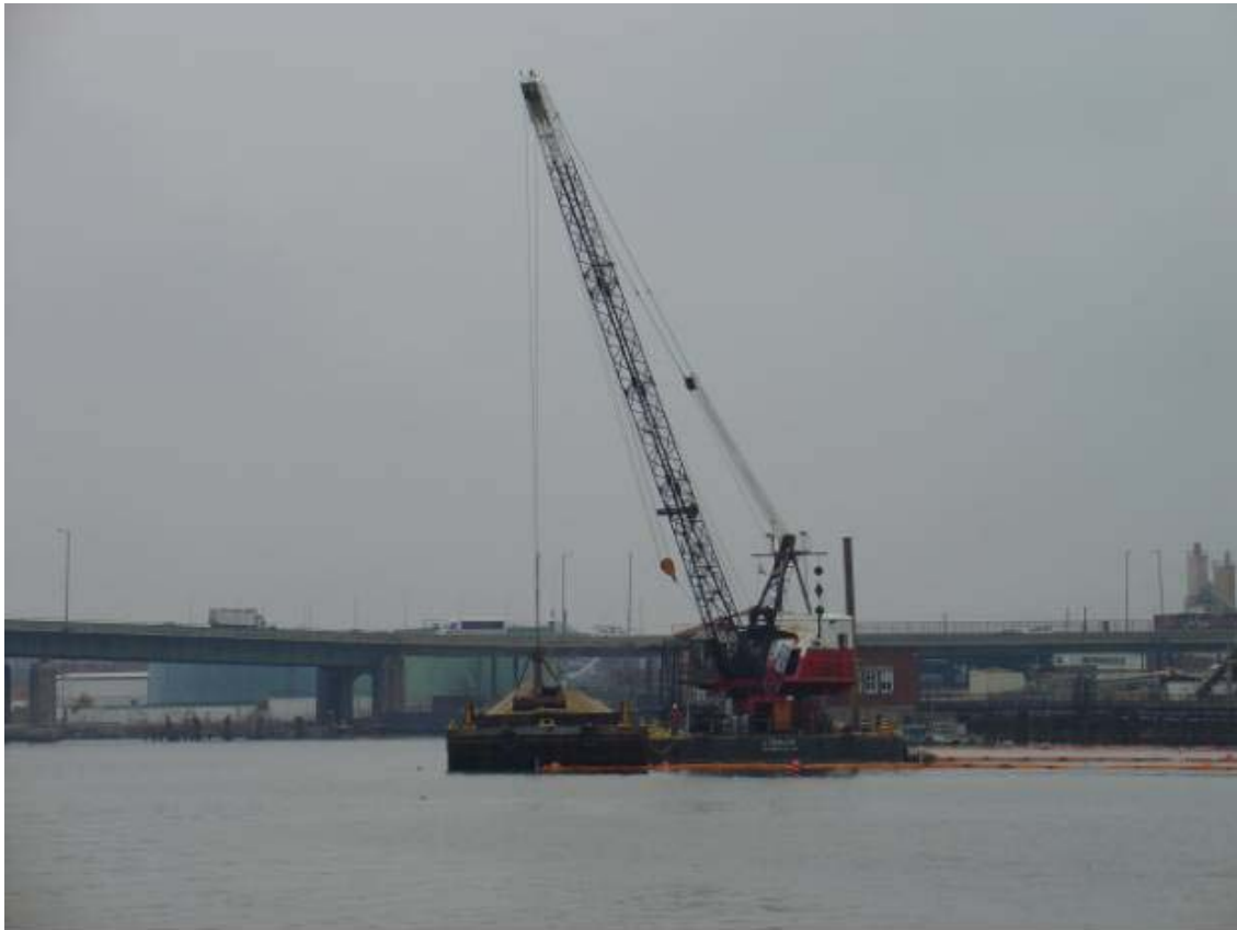
Figure 3-8. Crane Barge Used to Place Caps in Demonstration Area
