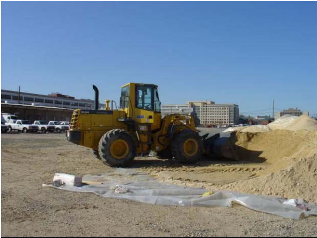
Figure 3-6. Sand Cap Material Stored in Bulk at Staging Area
