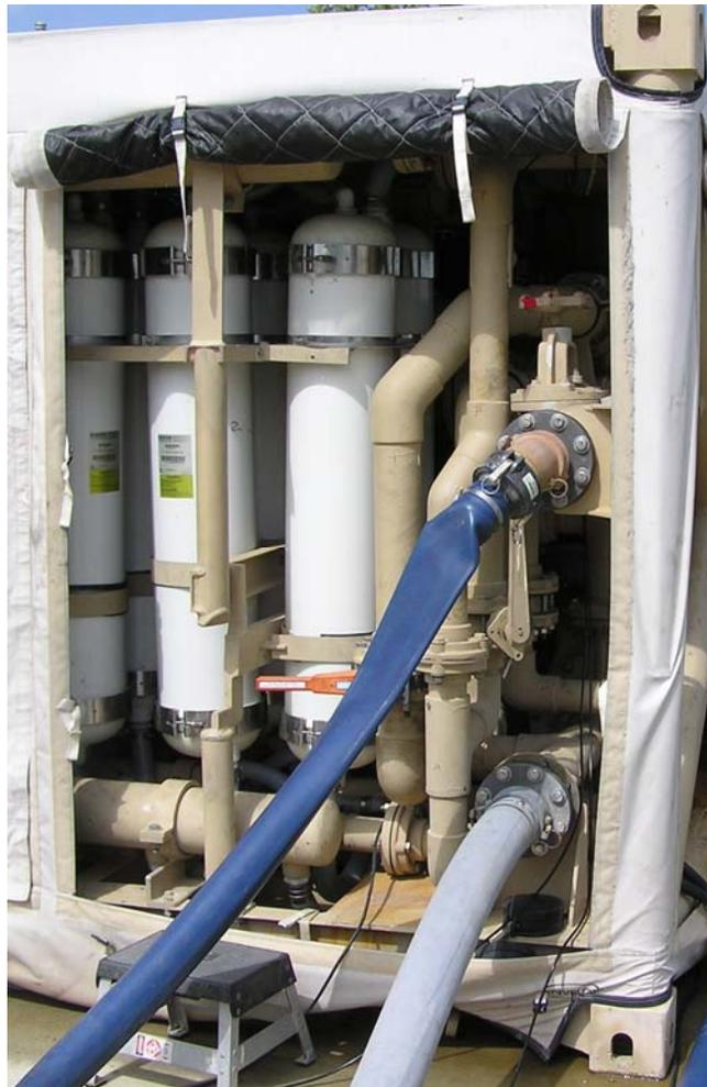
Figure 2-1. UF modules in the EUWP UF skid.
