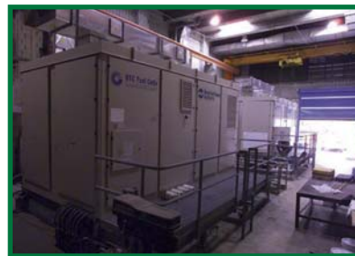
UTC fuel cells at wastewater treatment plant test site in Brooklyn
