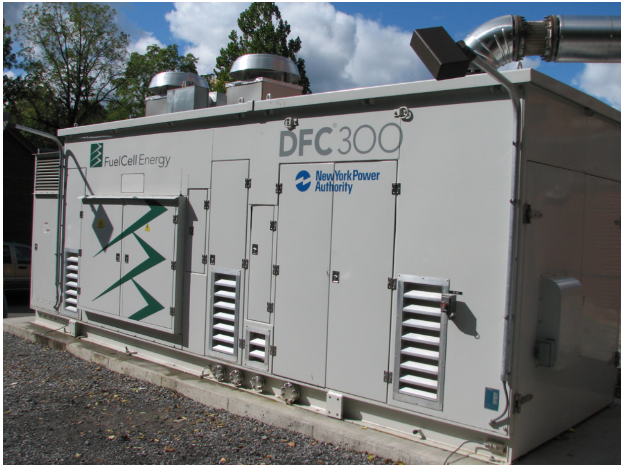
Figure 1-1. The FuelCell Energy DFC 300A at SUNY-ESF
