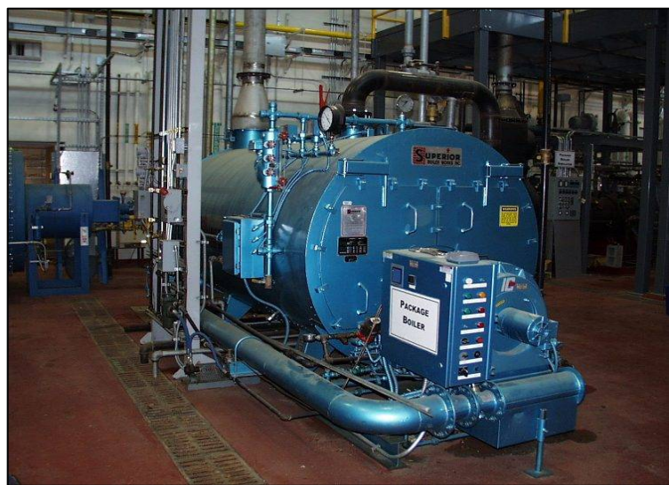
Figure 3-1. Wetback Scotch Marine Package Boiler
