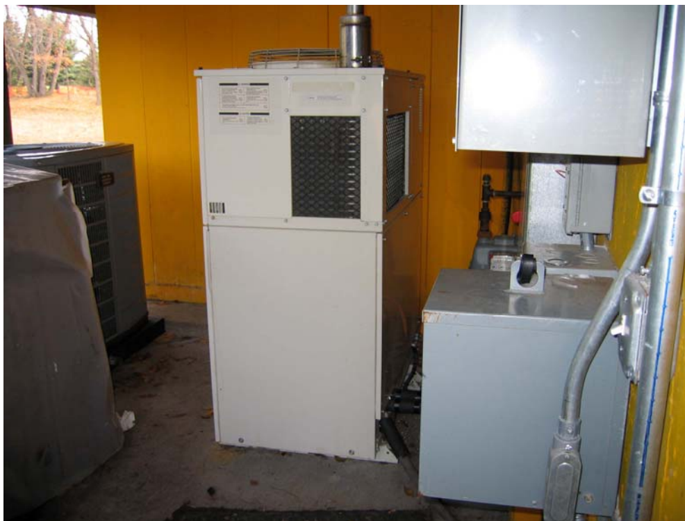
Figure 1-1. Current Installation of Aisin G60 Cogeneration Unit at Hooligans
