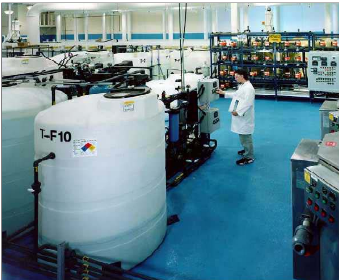
Photo 1. Aero-Electric Connector, Inc. facilities in Torrance, California, showing installation of Hydromatix 786E Ion Exchange treatment system and associated equipment.
