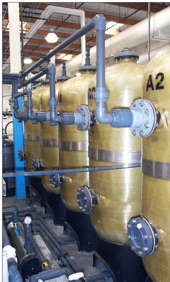
Photo 3. Ion exchange columns - 6' tall.
