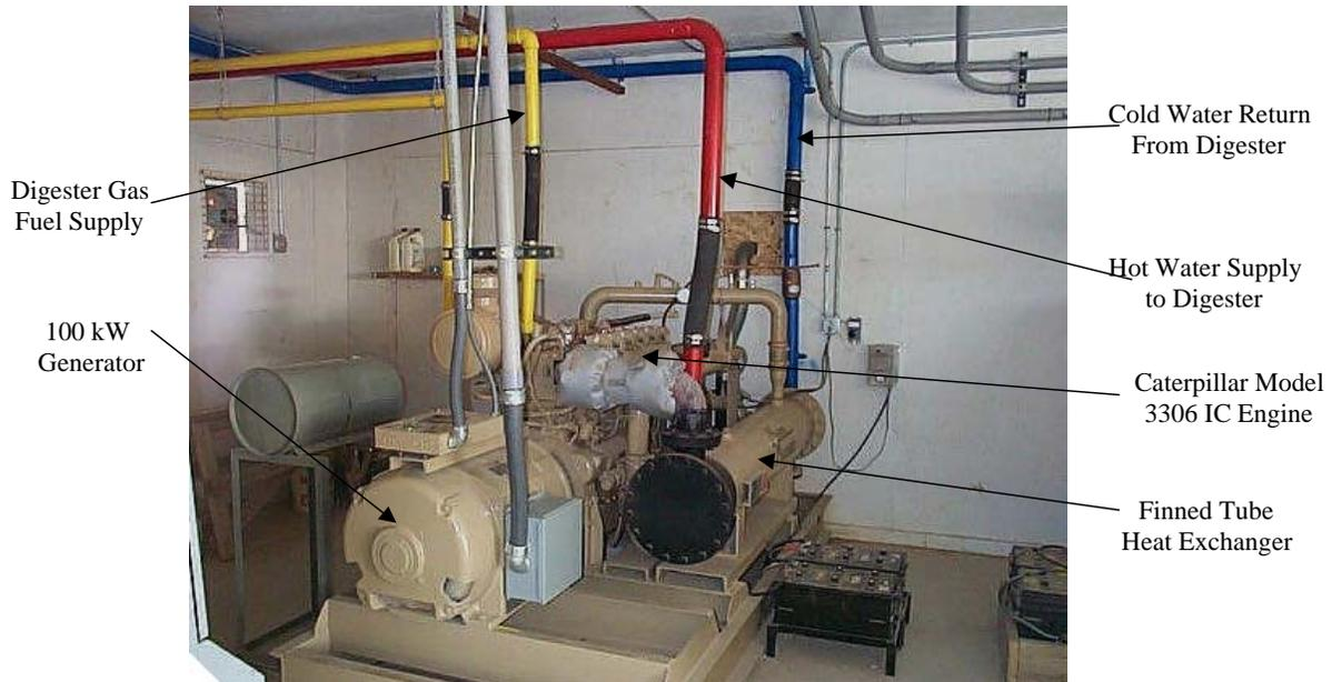
**Figure 1-1. The Colorado Pork IC Engine CHP System**
