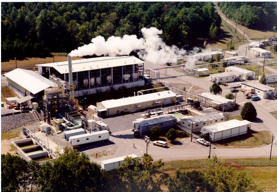
Figure 3-2. Overview of TSCAI Test Location. The incinerator stack is at left, with waste feed area behind the stack. The trailers housing the mercury CEMs for this test were located in the foreground at the base of the stack.
