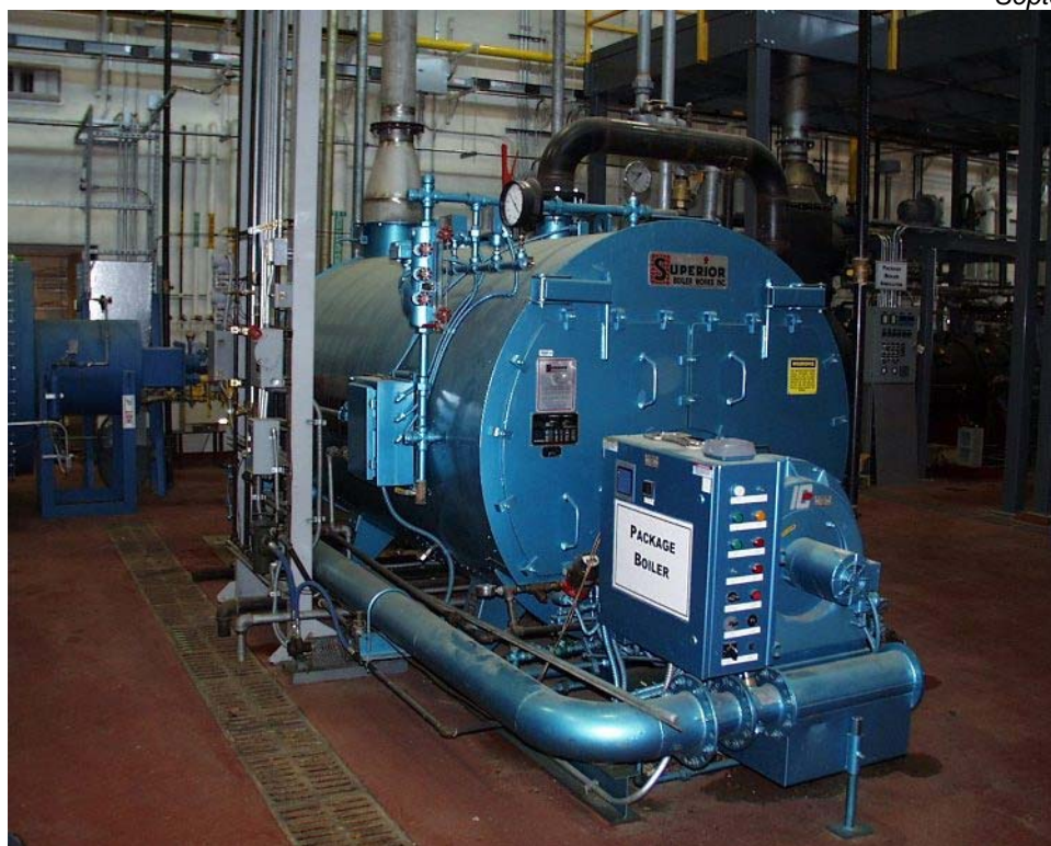
Figure 1. Wetback Scotch Marine Packaged Boiler
