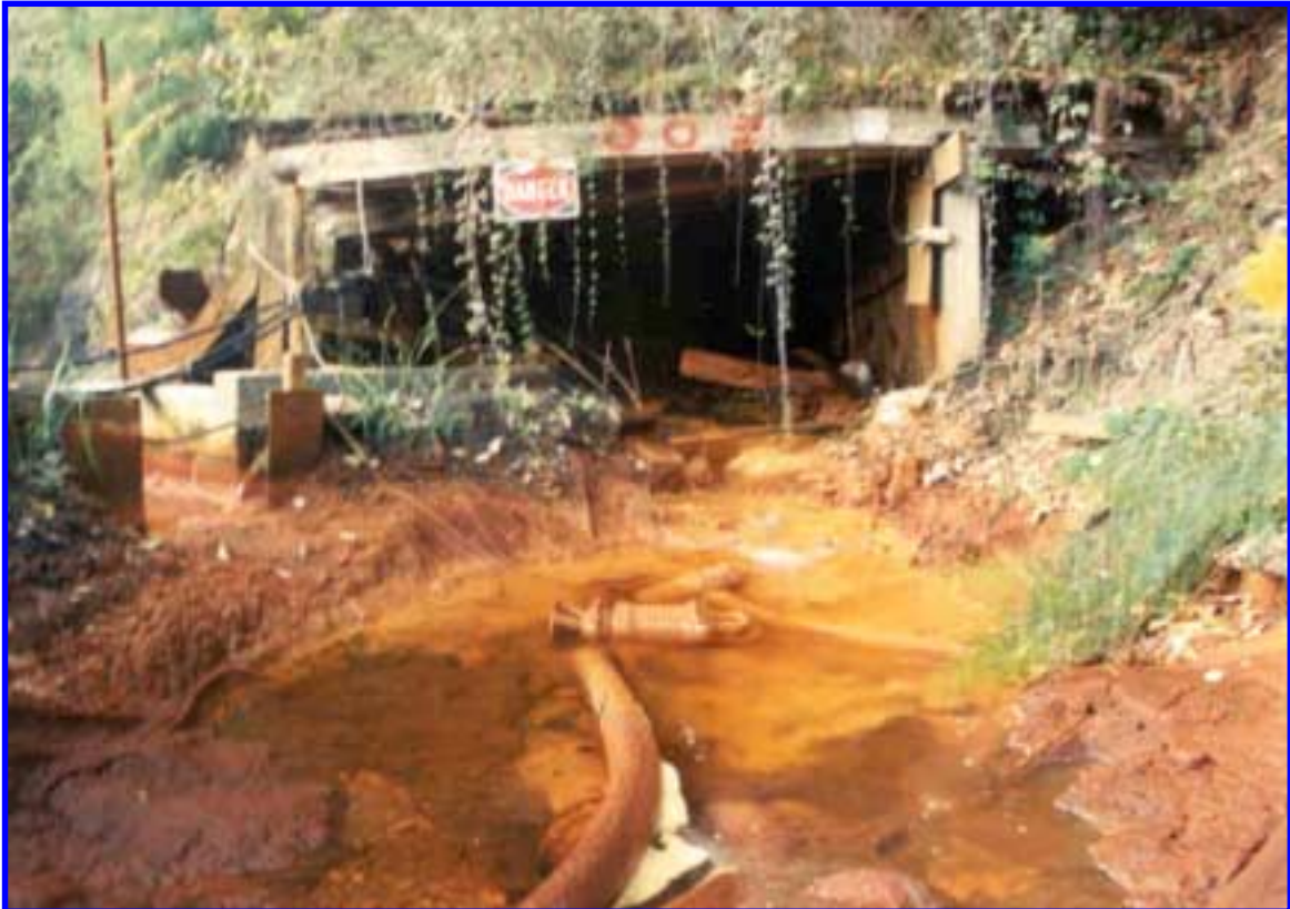
Acid Mine Drainage Flowing From Portal of T & T Mine on Sovern Run Cheat River Watershed
